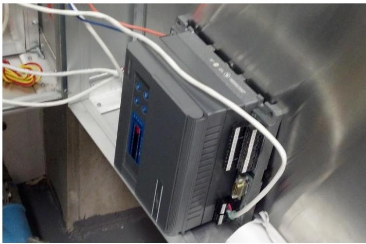
Figure 4.8 Additional DX controller responsible for sending signal to the FFD
