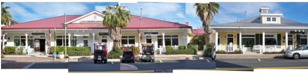
Figure 3-9. The Villages, Block C, East
