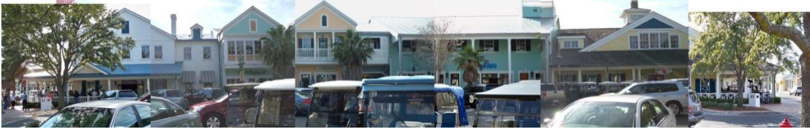
Figure 3-12. The Villages, Block E, West
