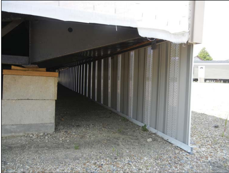
Figure 4.25 Up-Close View of Mobile Home Skirting
