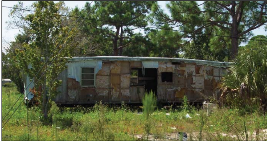
Figure 4.14. Abandoned Mobile Home, Source: Keef59, Flickr.com Used with permission.
