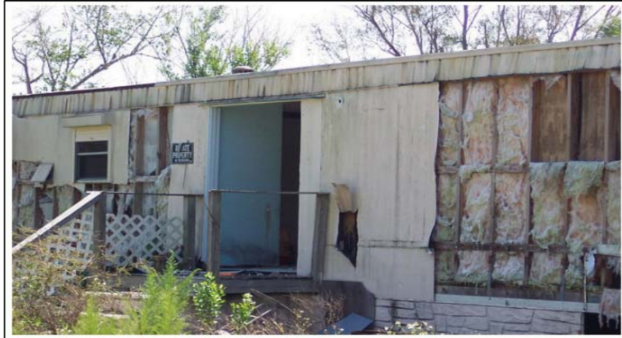
Figure 4.13 Abandoned Mobile Home, Source: Keef59, Flickr.com Used with permission.
