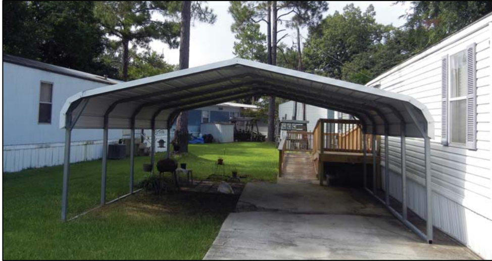
Figure 4.28 Carport and Patio Pavers
