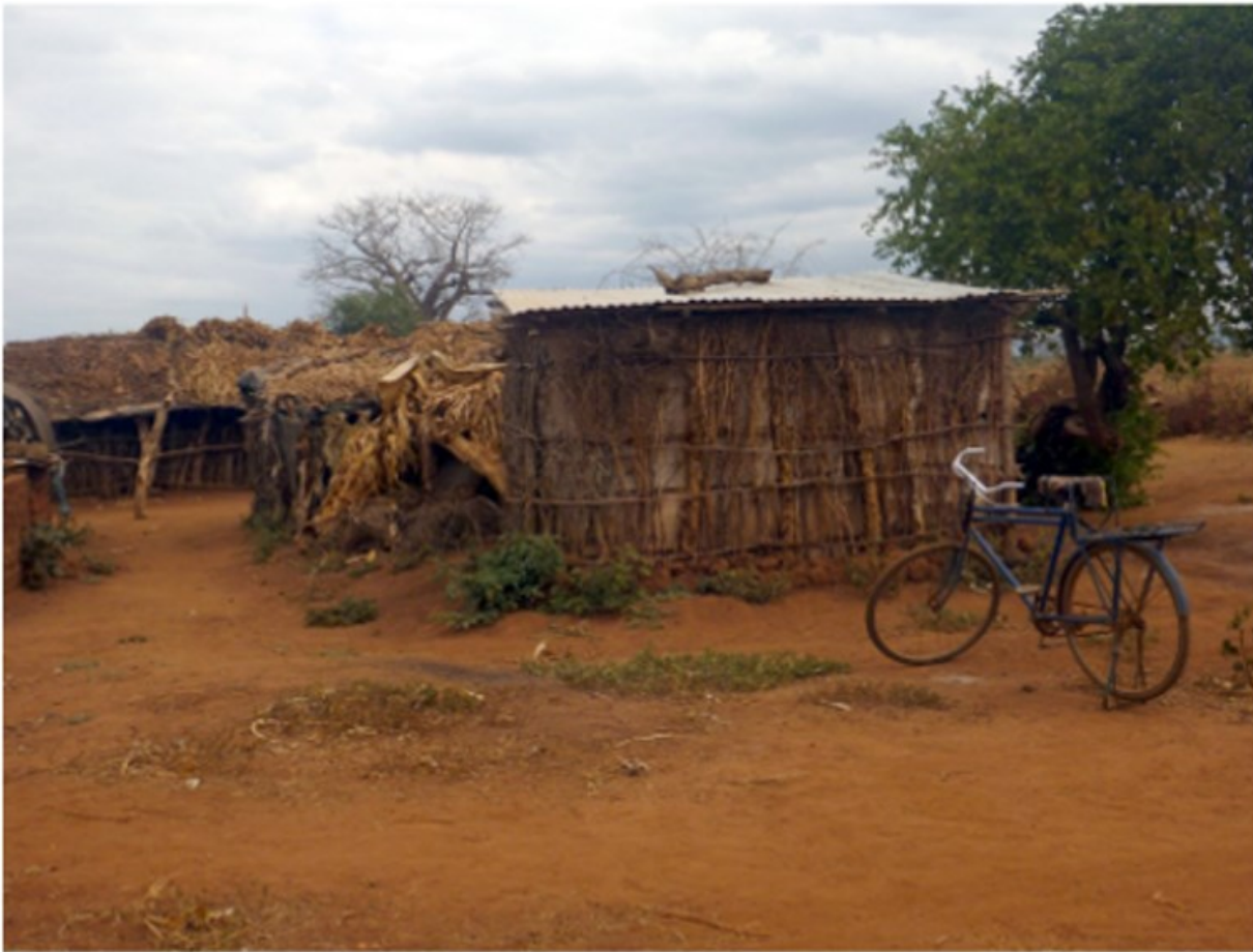
Figure 14. A squatter dwelling near the eastern boundary of Chyulu Hills National park. Photo taken on June 12, 2015.
