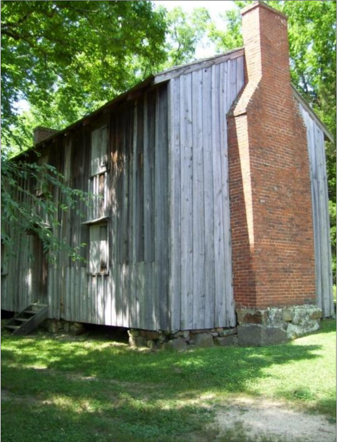
Figure 44. Outside of one of the slave quarters at Stagville plantation.
