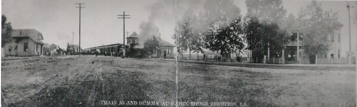
Figure 4.5b: Undated photograph of Baton Rouge Junction. The caption reads, “ Baton Rouge Junction Train 53 and Dummy in front of Baton Rouge Junction Depot People’s Hotel on left, and the first T & P Hotel on right.” (Courtesy of the Addis Historical Museum)
