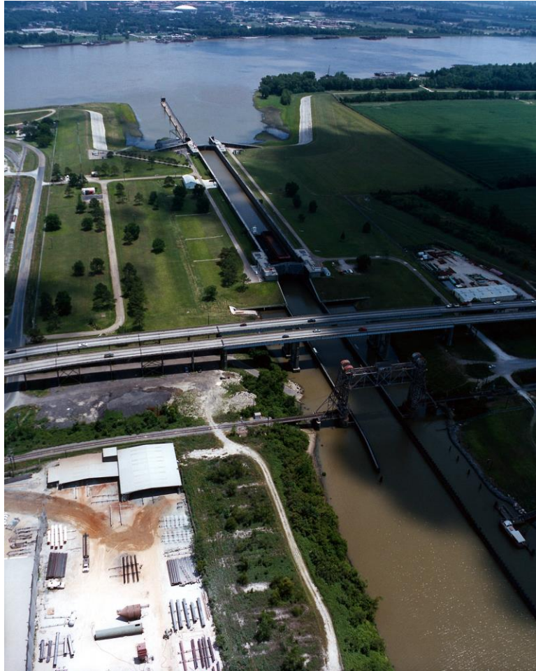
Figure 4.9: An aerial view of the Port Allen Lock looking to the east. (Courtesy of the U.S. Army Corps of Engineers)
