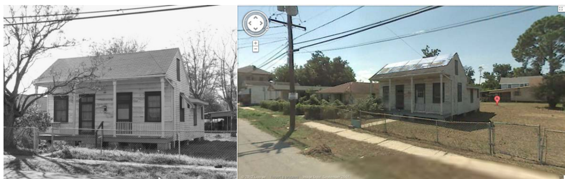
Figure 4.2: 832 Flood Street in 2002 and again in 2007 27
