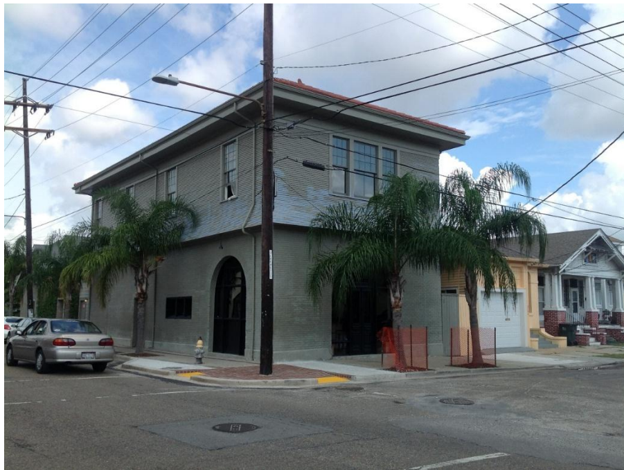
Figure 19. Building along Freret Street being renovated by Axel's Crew (2009).
