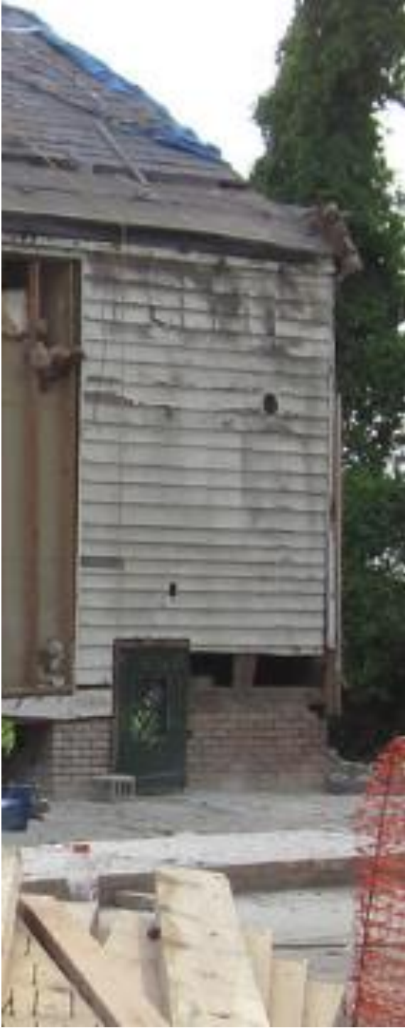
Figure 24 – Exterior of the raised cabinet and the cave
