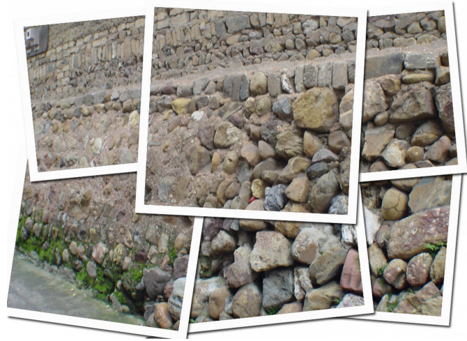
Figure 27 the texture of the Curtain Wall of the Old City, the layers showing construction efforts of different historical periods; source: photographed by Qiu, Xingjie and processed by author
