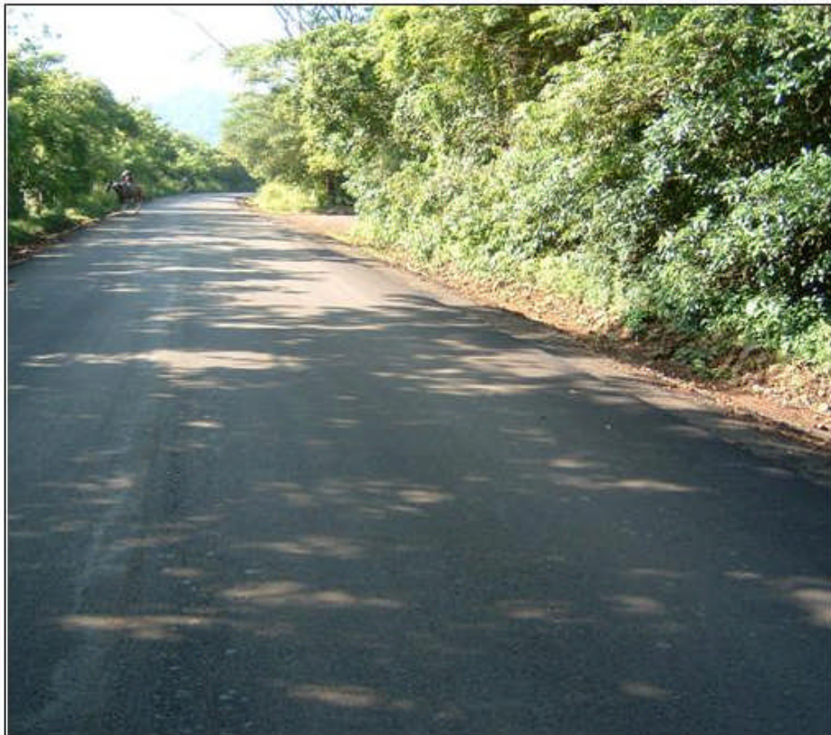
Figure 7.2: Main access road into region after paving
