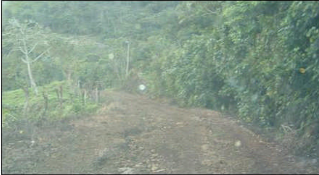
Figure 7.1: Main access road into region prior to paving
