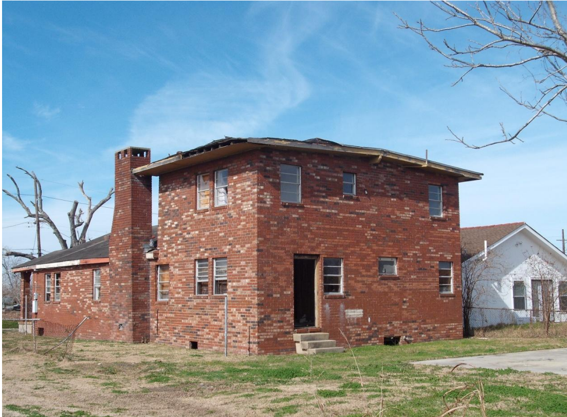
Figure 51. Abandoned home in Plum Orchard (photo by author)
