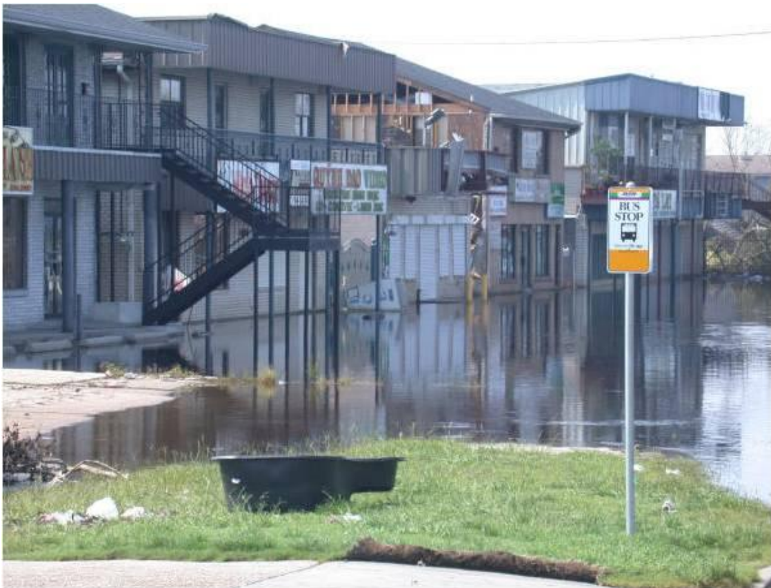
Figure 44. Damaged Alcee Fortier Blvd. Strip Mall (photo by MQVNC)
