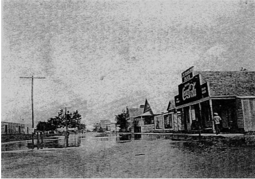
Figure 20: Floodwaters inundating downtown Morganza
