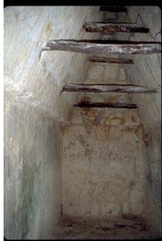
Figure 1-4: Wooden beams inside a corbelled vault of Structure 5D-65 in the Central Acropolis of Tikal, Guatemala. Photograph by Linda Schele, David Schele, reprinted with permission of Foundation for the Advancement of Mesoamerican Studies, Inc., www.famsi.org .
