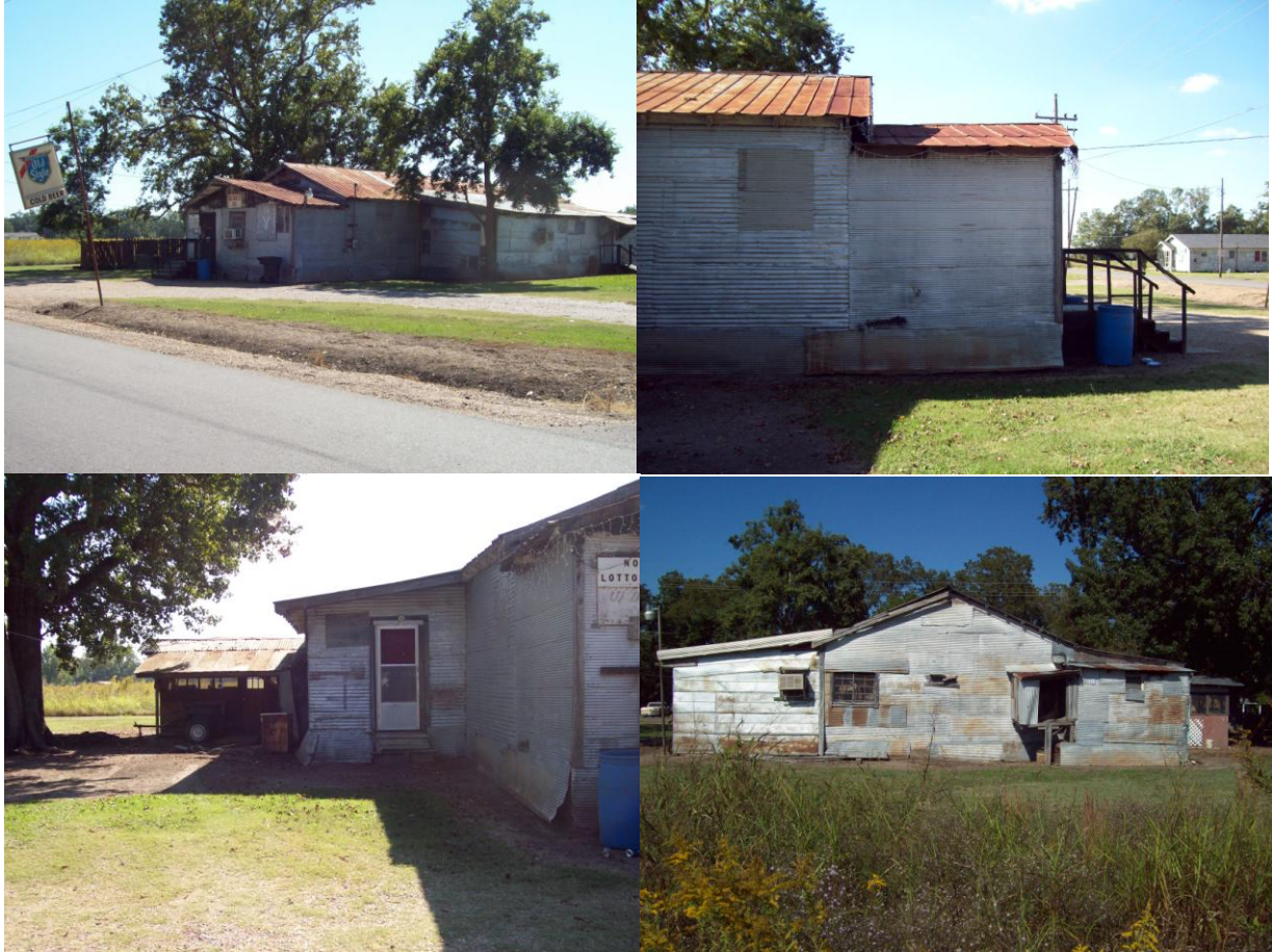
Figure 4-2: Exterior Photographs Showing the Additions to the Disco 86 Lounge (Source: Author)
