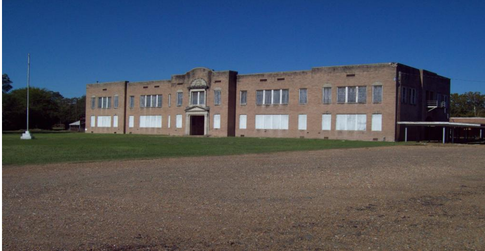
Figure 3-4: Abandoned Waterproof High School Building, 2008 (Source: The Author)
