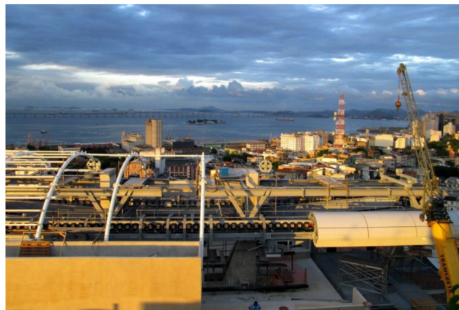
Figure 5.3 Construction of the teleférico . Photo taken by author, 2013.
