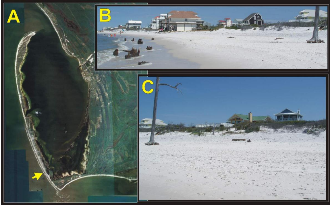
Figure 5.57 – Profile R100. Photo A marks the location of the profile in Gulf County, Florida. Photo B looks north along the eroding shoreline. Photo C displays the foredune and development landward of the foredune crest.
