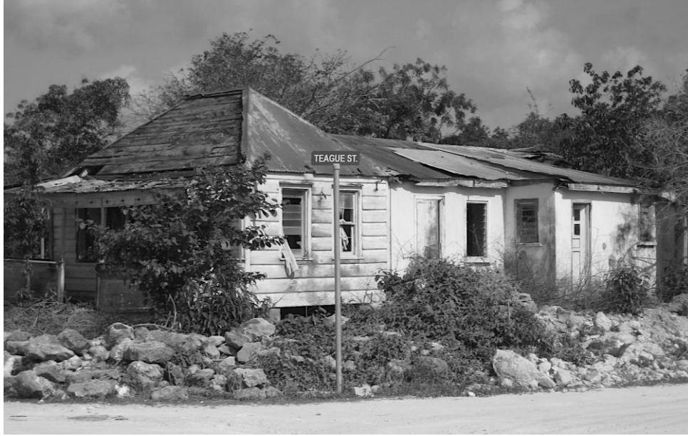
Figure 2.6 Dilapidated Home in Codrington Village
