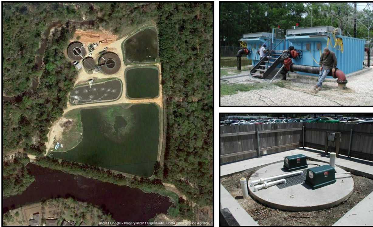
Figure 1.3 Wastewater Plants, Regional Plant (left) Smaller Plants (right) (Google 2011).
