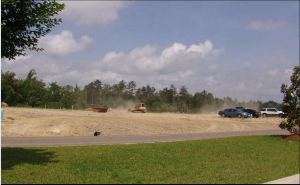
Figure 2.2 Urban Development (with no BMPs) on Hwy 21, between Hwy 190 and I-12 in the Tchefuncte Watershed (western St. Tammany) (2011).
