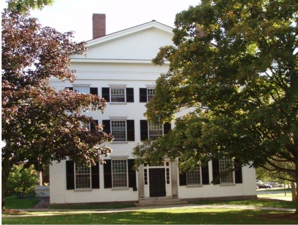
Figure 19: Reed Hall. Photo by author.
