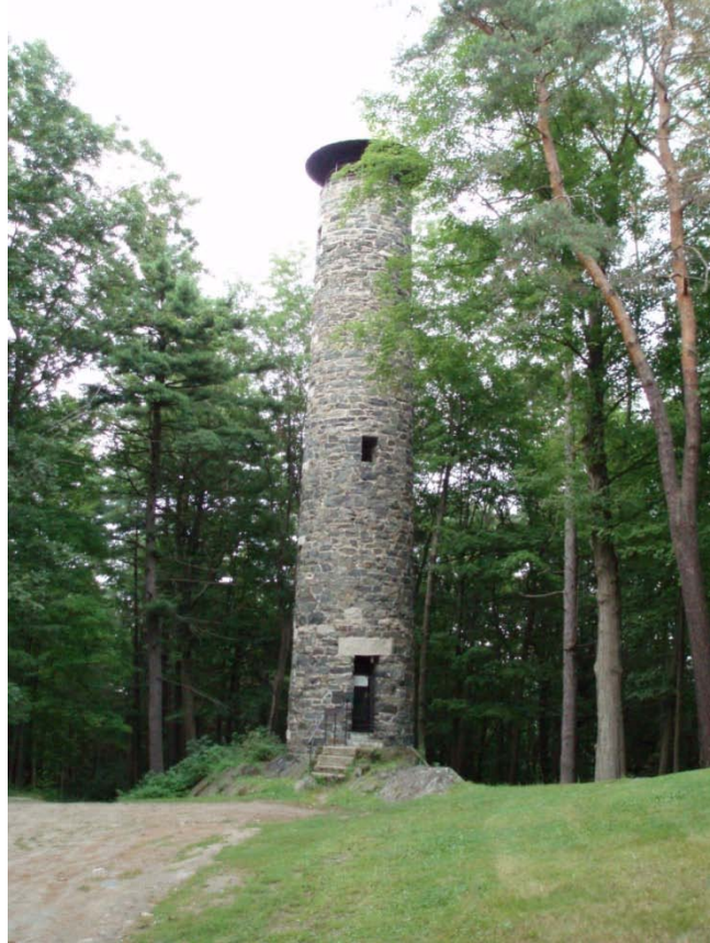
Figure 36: Bartlett Tower. Photo by author.
