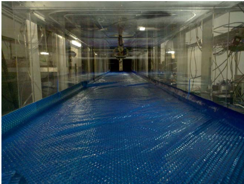
Figure 3.3. The insulating cover installed over the water surface.
