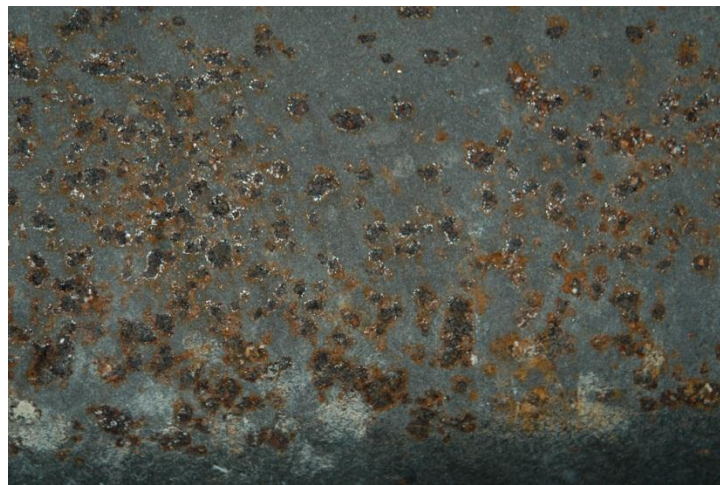
Figure 6 Pitting corrosion occurs on the surface of cast iron bathtub (Courtesy J.E.I. Metallurgical Inc)
