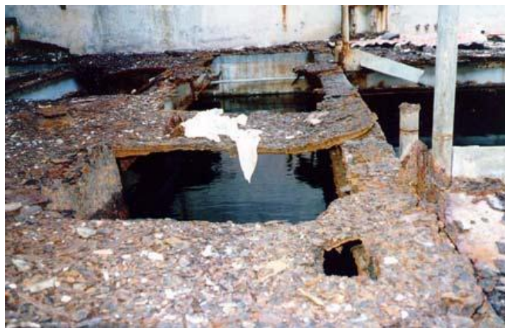
Figure 3 Uniform attack on the outside of water tank (Courtesy NASA Corrosion Technology Laboratory)
