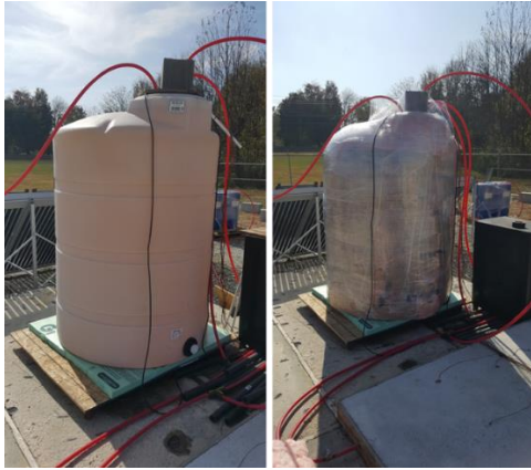
Figure 35: Filling and insulating the aboveground storage tank.
