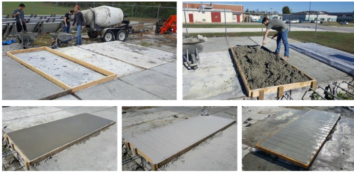
Figure 28: Electrical system concrete slab construction.
