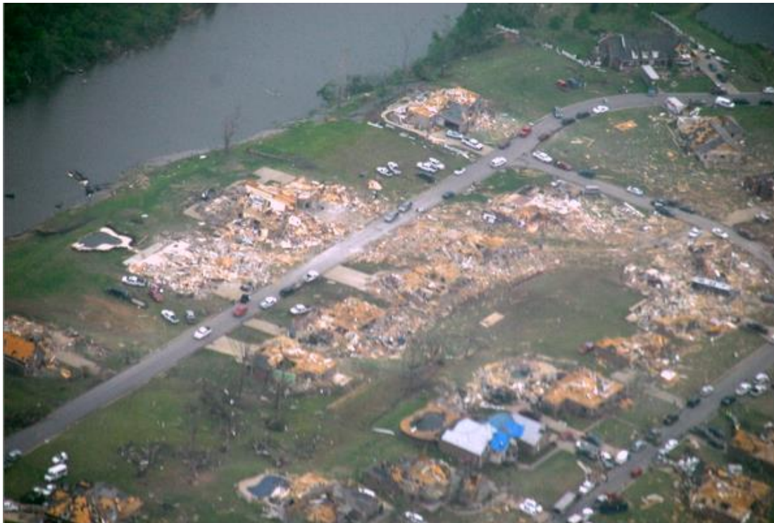
Figure 5.10 Severe damage in a neighborhood at location (R2L1) rated as EF4, taken by CAP (2014).
