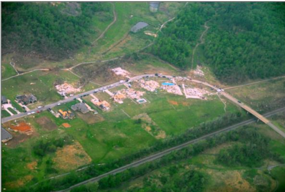
Figure 5.12 Severe damage in a community at location (R2L2) rated as EF4, taken by CAP (2014).
