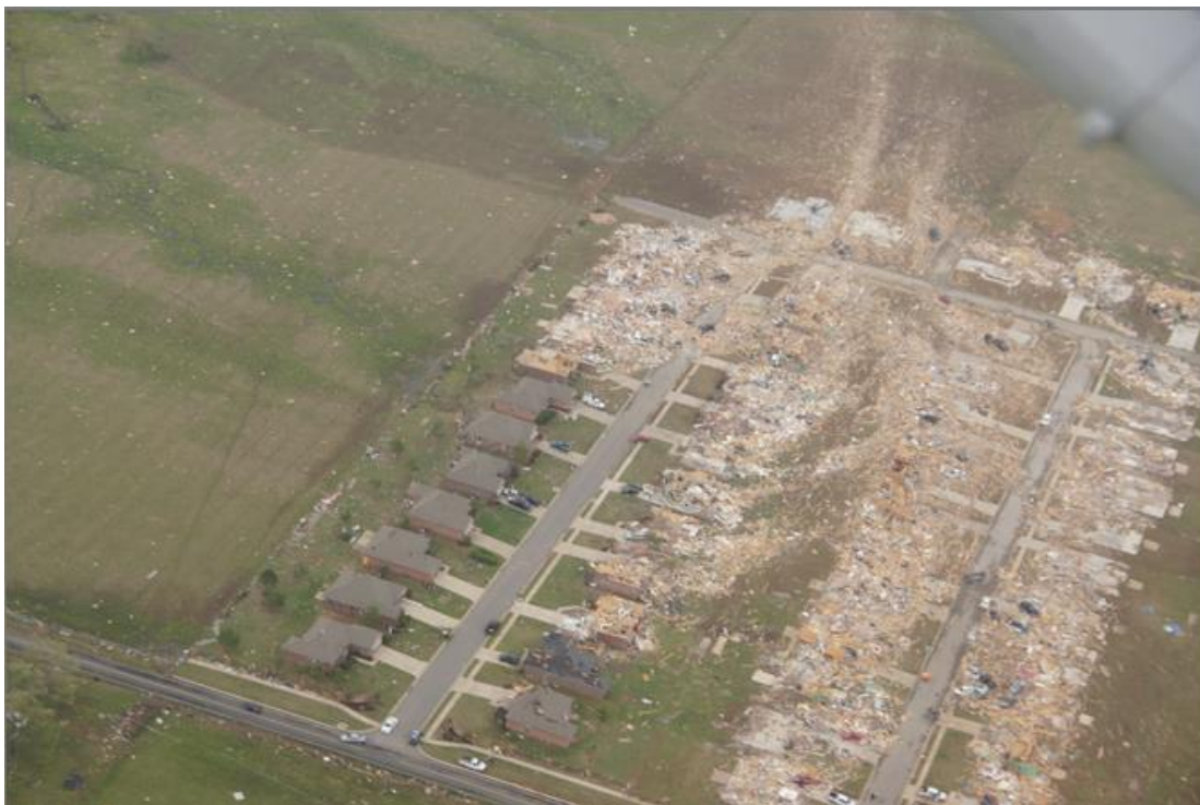
Figure 5.29 A neighborhood in Vilonia (R4L2) almost completely grounded, Taken by CAP (2014).
