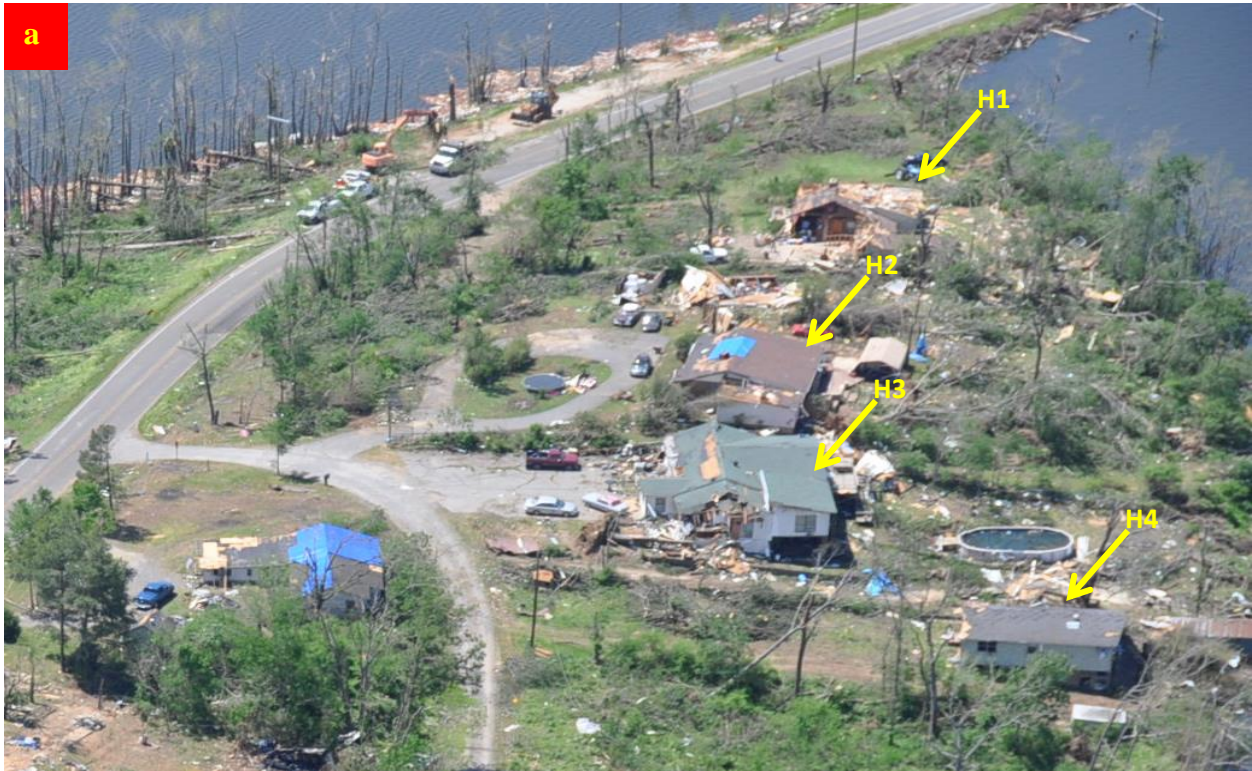
Figure 4.19 a) Aerial view taken from the east side for house (H1-H4) taken from CAP (2014).
