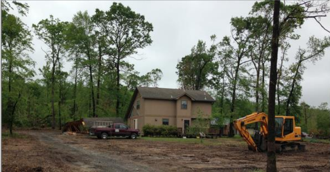
Figure 5.5 A house in location (R1L1) with a damage rating as EF1, only the shade attached to the house is collapse, taken by UA team.
