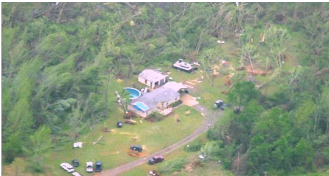
Figure 5.19 Damage in residential house rated as EF2, R3L1 taken by CAP (2014).
