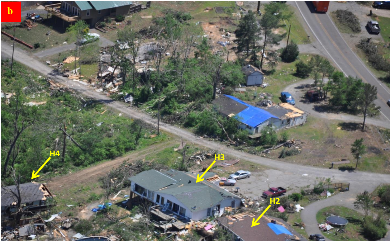
Figure 4.20 b) Aerial view taken from the west side for house (H2-H4) on the leeward side (low elevation, less damage EF1) taken from CAP (2014).
