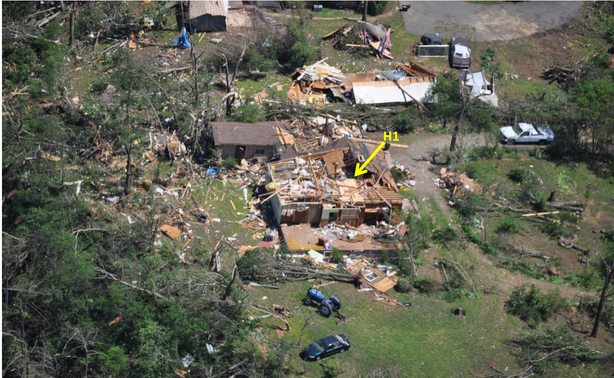
Figure 4.18 Aerial image for a severe damage for house (H1) uphill (Source CAP, 2014).
