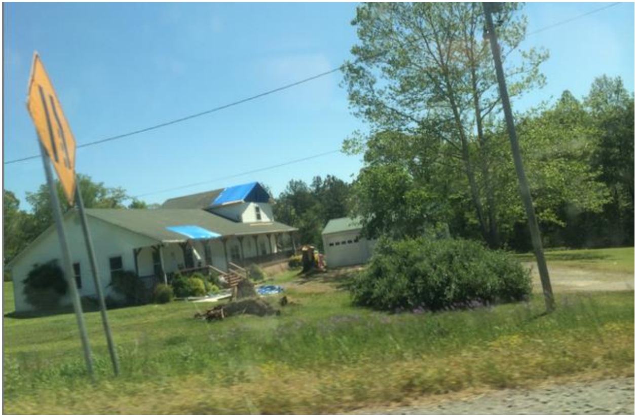
Figure 5.31 Minor damage observed at the house in location R4L3, taken by UA team.
