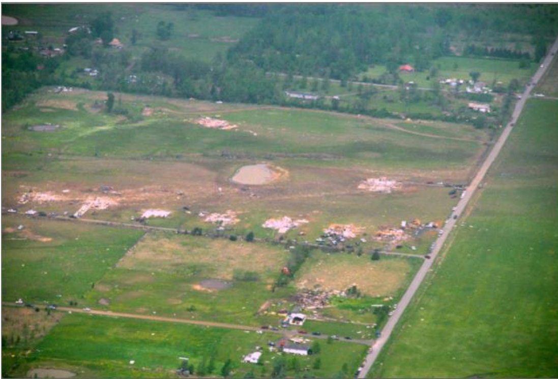
Figure 5.23 A whole community destroyed due to tornado right before Vilonia bypass at R3L2.
