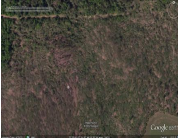
Figure 2.18 Tornado damage, while traveling up the hill (Selvam & Ahmed, 2013).
