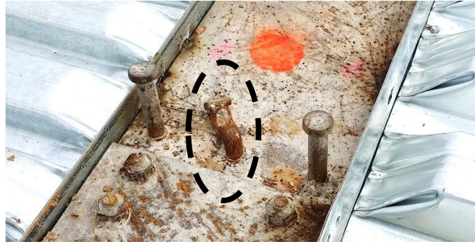
Figure 50 showing shear stud bend to a 90 degree angle as a result of being hit with a jackhammer during concrete removal. Shear stud is still attached firmly to the steel flange
