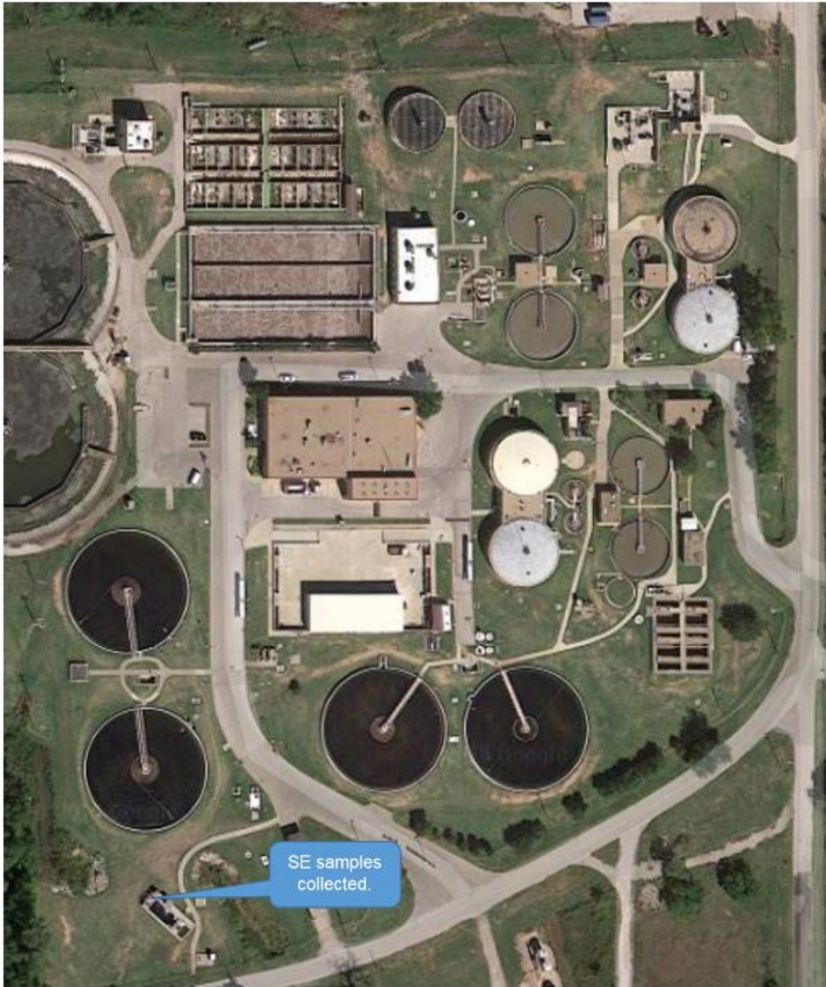
Figure 3-6: COK WRRF Site Aerial (Google Maps)
