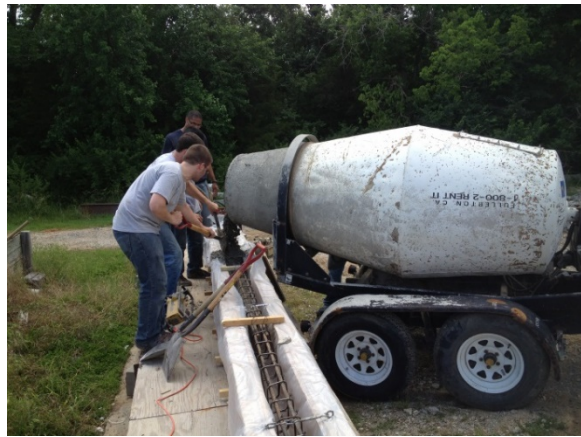
Figure 3.7 – Casting concrete.
