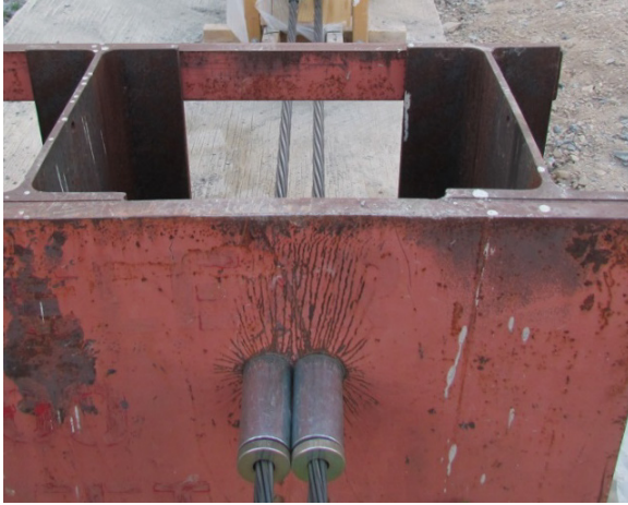
Figure 3.4 – Anchor prestressing strand using chucks (dead end).
