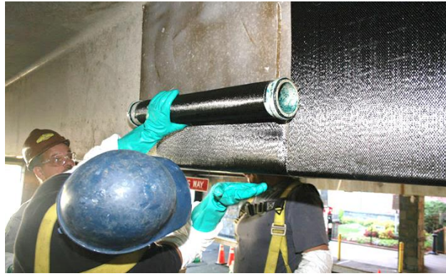
Figure 12. Bonded CFRP strips used to strengthen concrete structure (Alkhrdaji, 2015)
