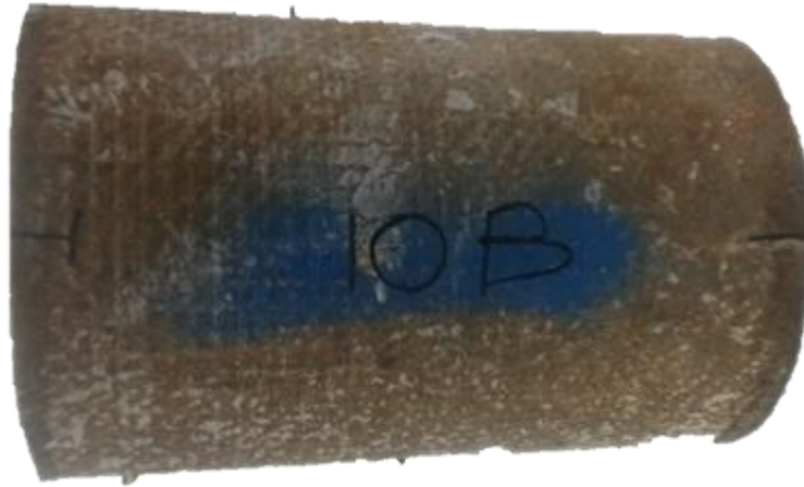
Figure 5-1. Sample 10B depicting the external surface of AC pipe
