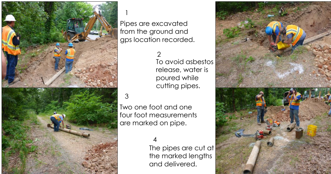
Figure 3-3. AC pipe sampling procedure
