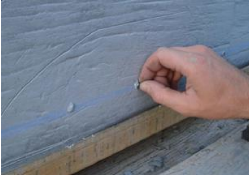
Figure 2-2. Placement of DEMEC points (Photo by author).
