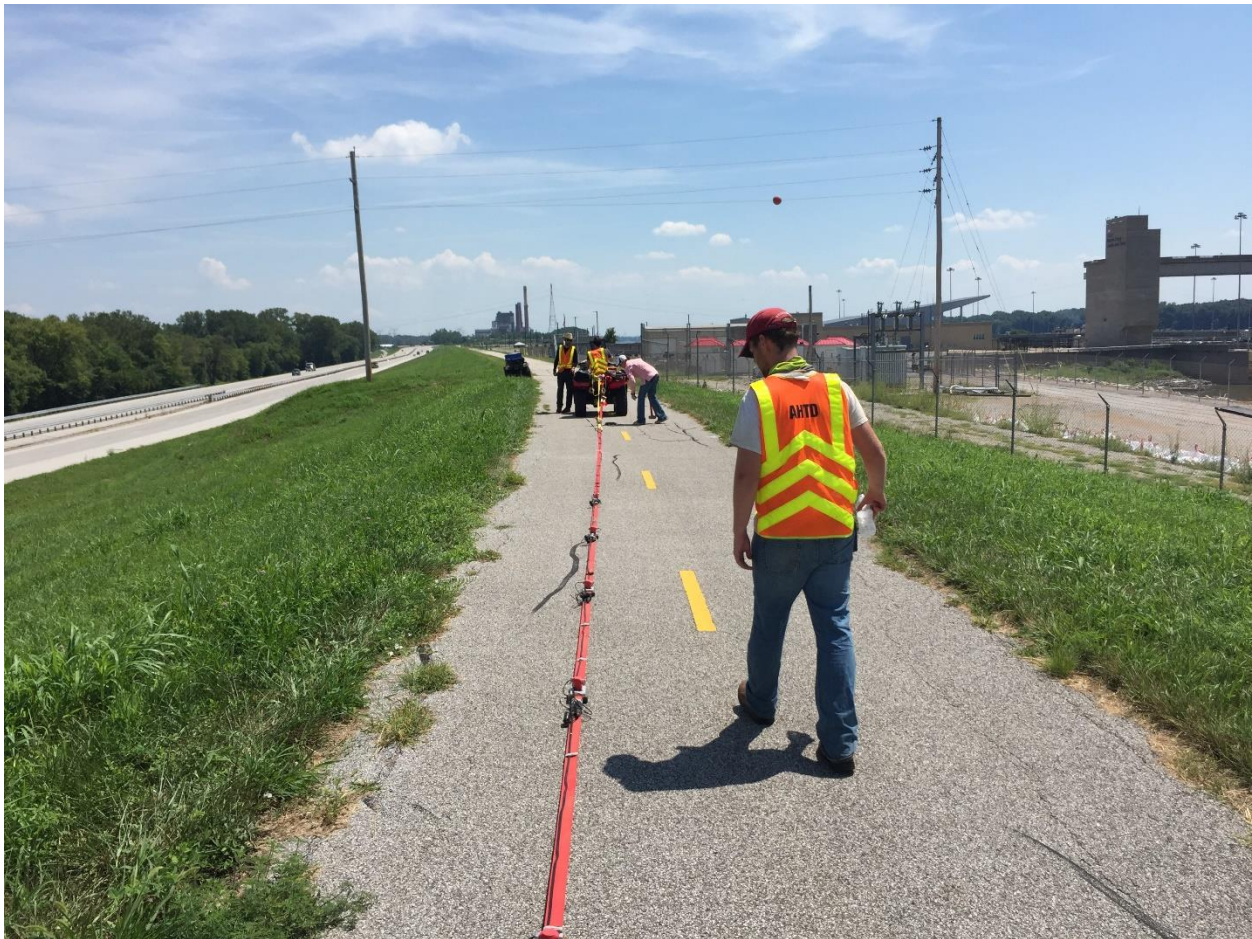
Figure 13 - Use of land streamer to collect seismic wave velocity data on top of a levee in Mel Price lock and Dam in Edwardsville, IL
