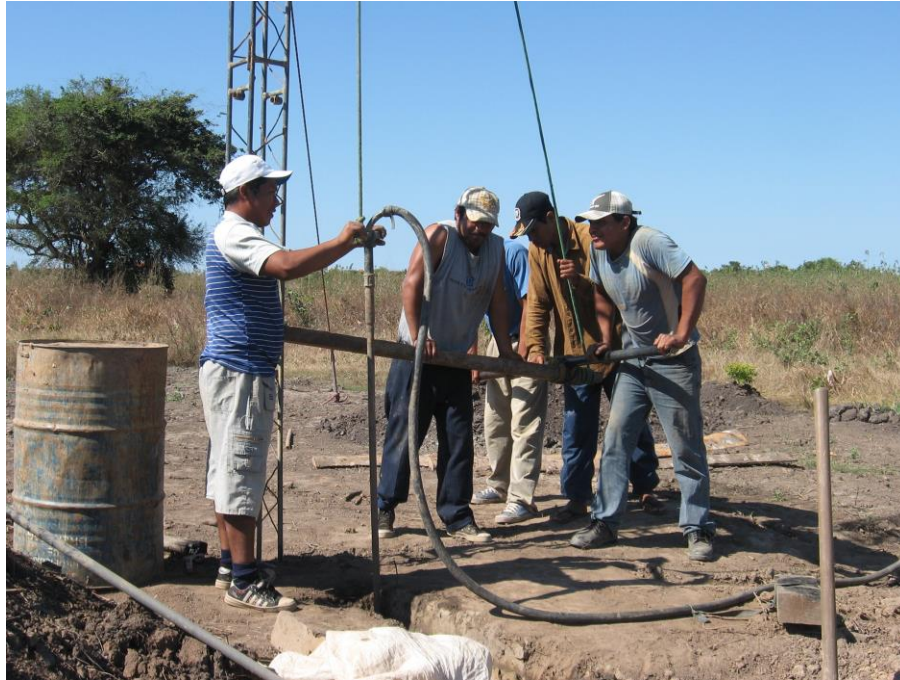
Figure 3-9. EMAS percussion-jetting-rotation manual drilling, Trinidad (Beni region)
