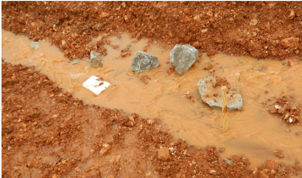
Figure 2.2: Photograph of the APS 703d type Floc Log roped around a stake. Photo taken by Bryan Signorelli (AHTD) on June 18, 2015.
