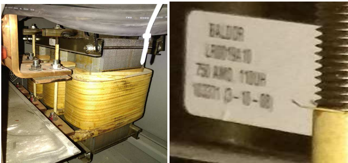
Figure B.6 Filter inductors in VVVF (left) and model of the filter Inductors (right).
