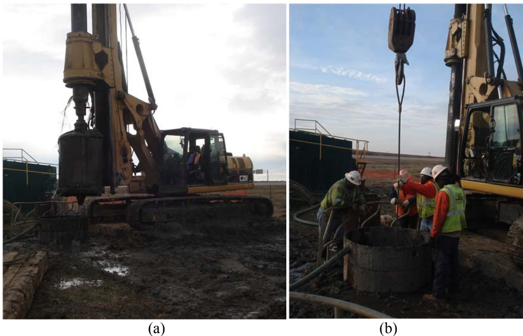
Figure 6.18. Photographs of (a) auger bucket during excavation, and (b) auger bucket retrieval.
