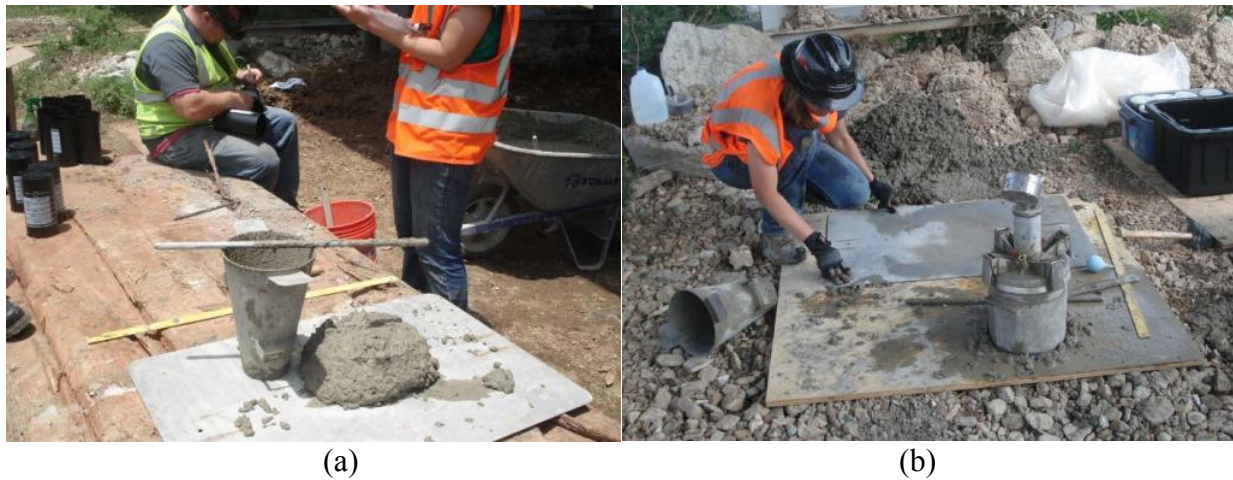
Figure 5.10. Photograph of concrete quality assurance testing including (a) slump and cylinder casting, and (b) air content testing.
