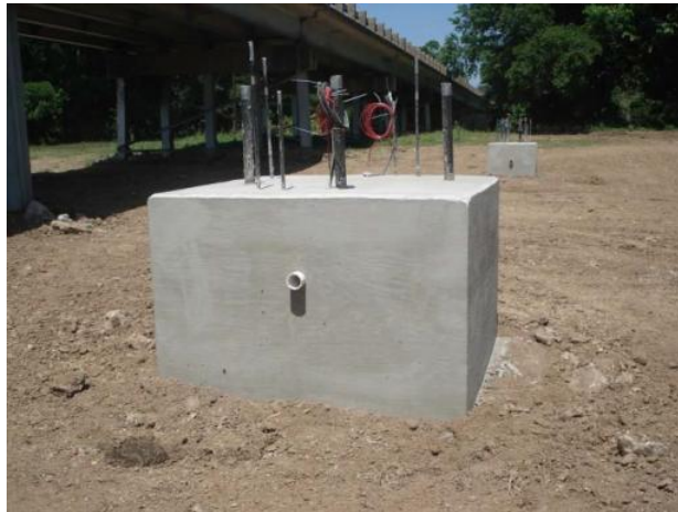
Figure 5.19. Photograph of the Test Shaft SS-C6 finished construction.
