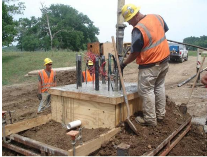
Figure 5.21. Photograph of Test Shaft SS-E4 four foot reveal construction.
