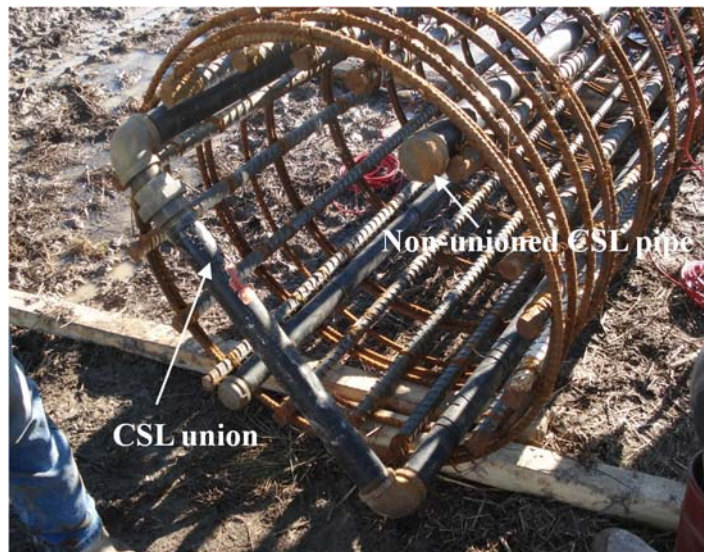
Figure 6.38. Photograph of CSL union at the bottom of the T-N4 reinforcement cage. A diagram of a completed top-down view and a photograph of the instrumented test shaft T-N4 are presented in Figure 6.39. Black tape on the end of the gauge wire indicated the “B” side of the shaft.
