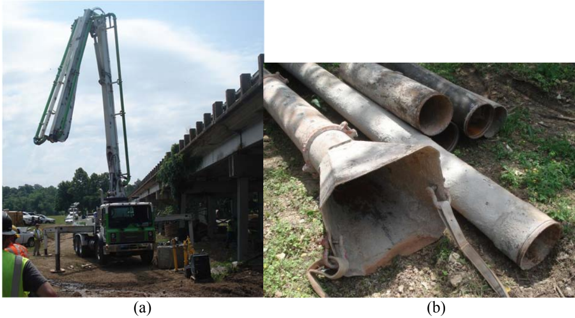
Figure 5.9. Photograph of the concrete placement equipment utilized during construction including the (a) Mantex R-232 concrete pump truck, and (b) tremie pipe.
