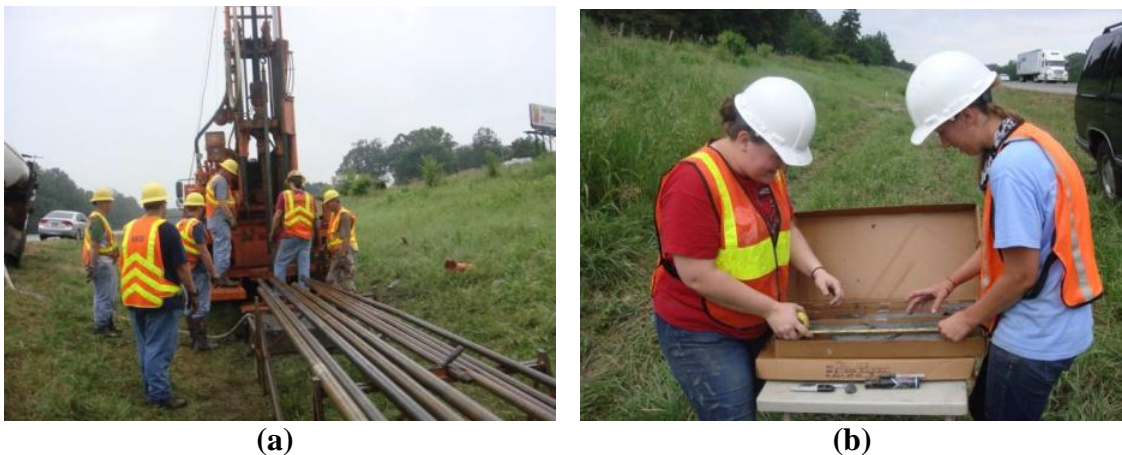
Figure 6.4. a) Drilling operations at B-3, and b) measuring RQD of rock sample obtained from B-3.
