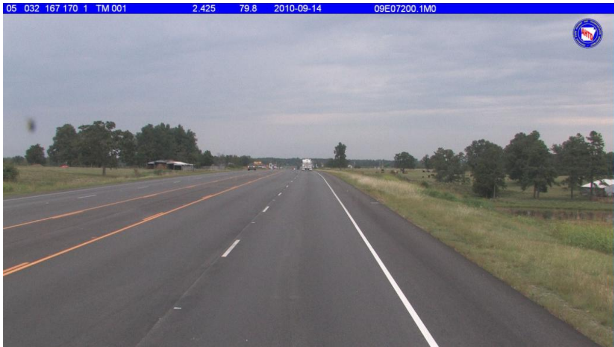
Figure 6.24 ROW of R50084 after resurfacing in September 2010
