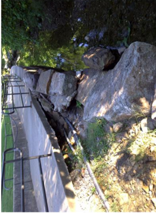
Figure 16b. Sidewalk area after 2009 repairs
