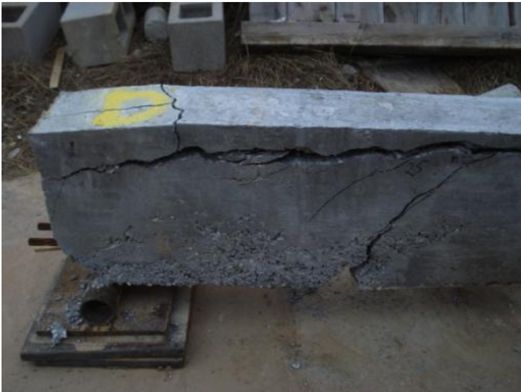
Figure 6.50: Shear cracking and failure of specimen NSL-4D
