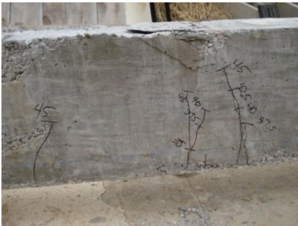
Figure 6.48: Cracking and failure of specimen NSL-3L
