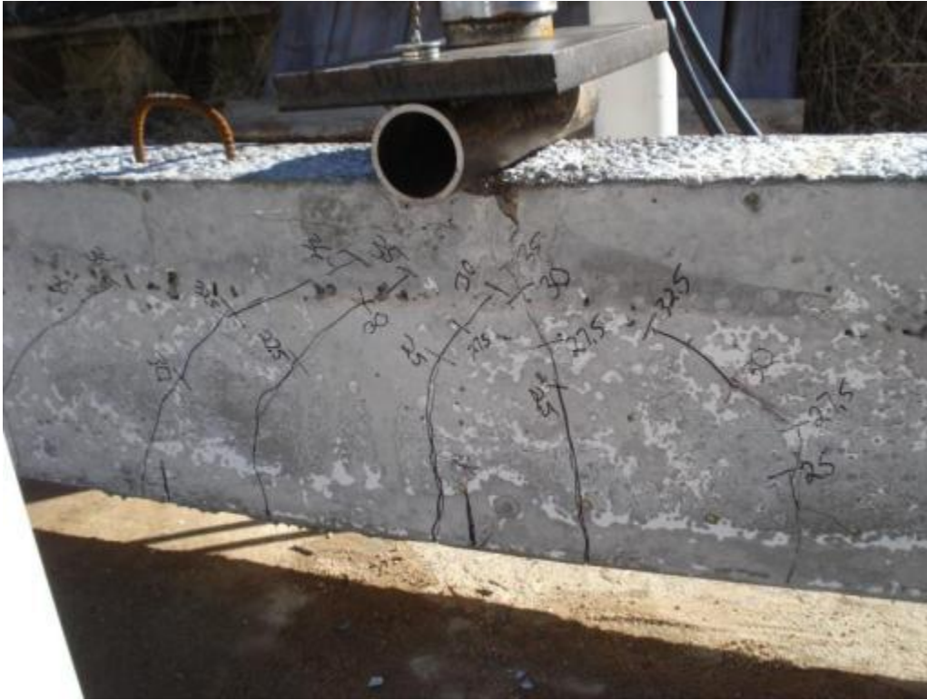
Figure 6.15: Cracking behavior of specimen NSC-4L
