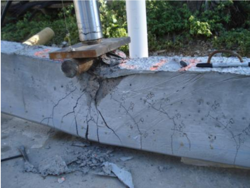
Figure 6.81: Cracking and failure of specimen HSS-4D
