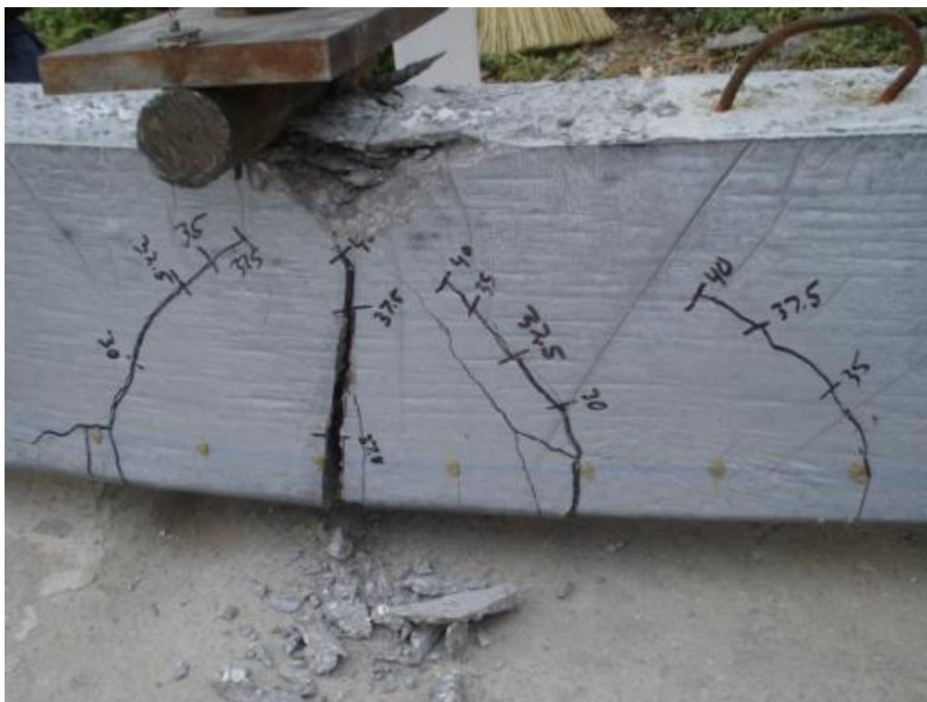
Figure 6.94: Cracking and failure of specimen HSL-3D
