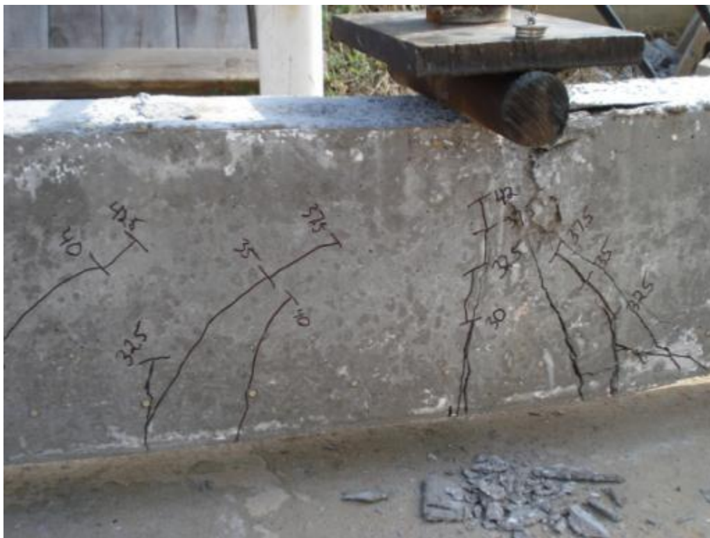
Figure 6.39: Cracking of specimen NSL-1L
