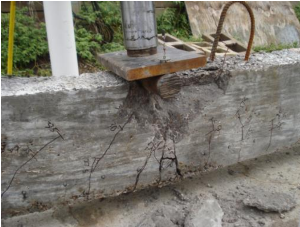
Figure 6.18: Cracking behavior and failure of specimen NSS-1D
