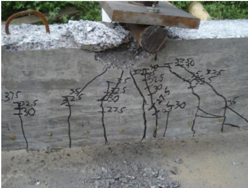
Figure 6.28: Failure of specimen NSS-3L
