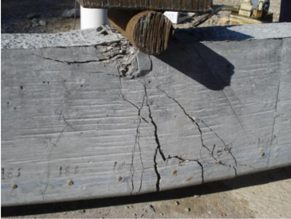
Figure 6.97: Cracking and failure of specimen HSL-4D
