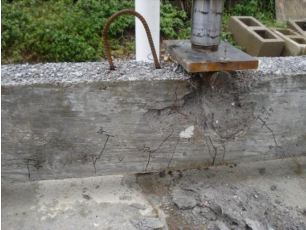
Figure 6.20: Cracking behavior and failure of specimen NSS-1L
