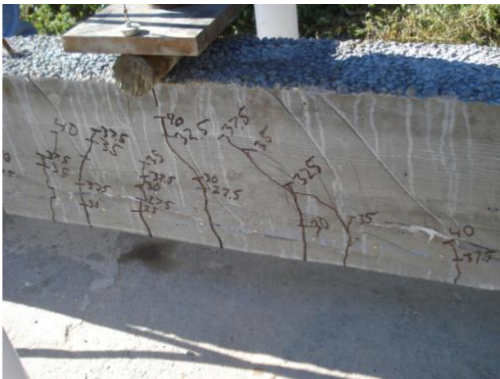
Figure 6.55: Cracking of specimen HSC-1L
