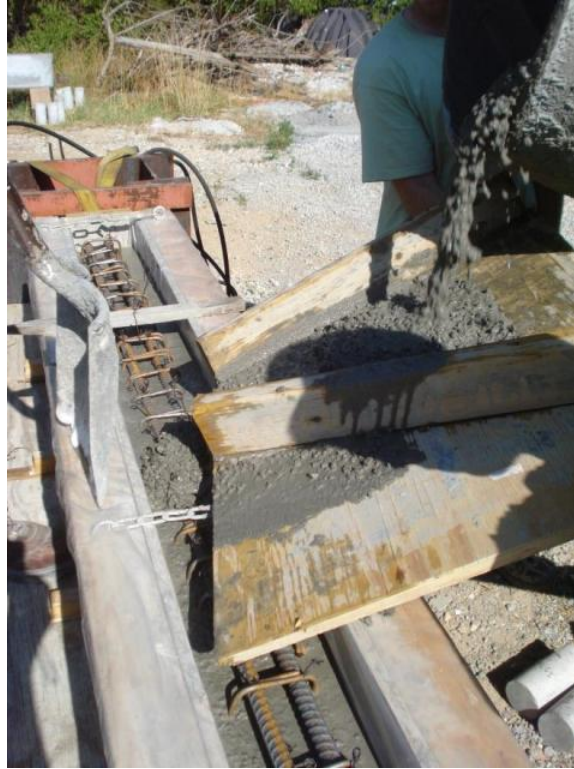
Figure 3.15: Concrete placement directly from the mixer
