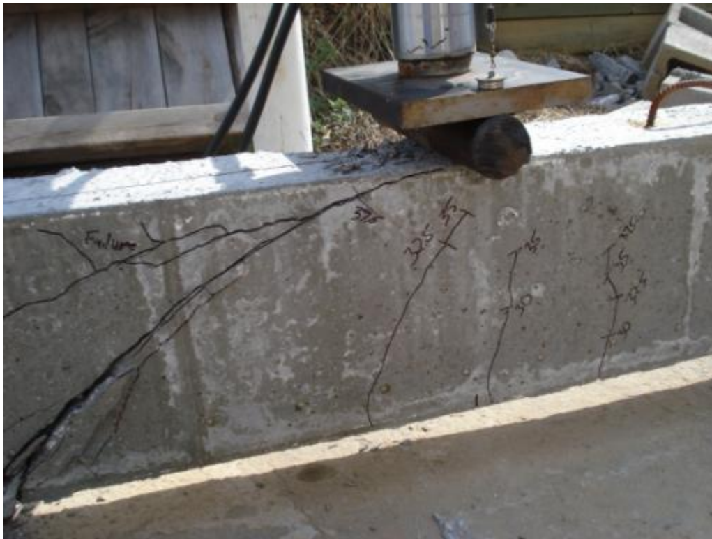
Figure 6.37: Shear cracking of specimen NSL-1D
