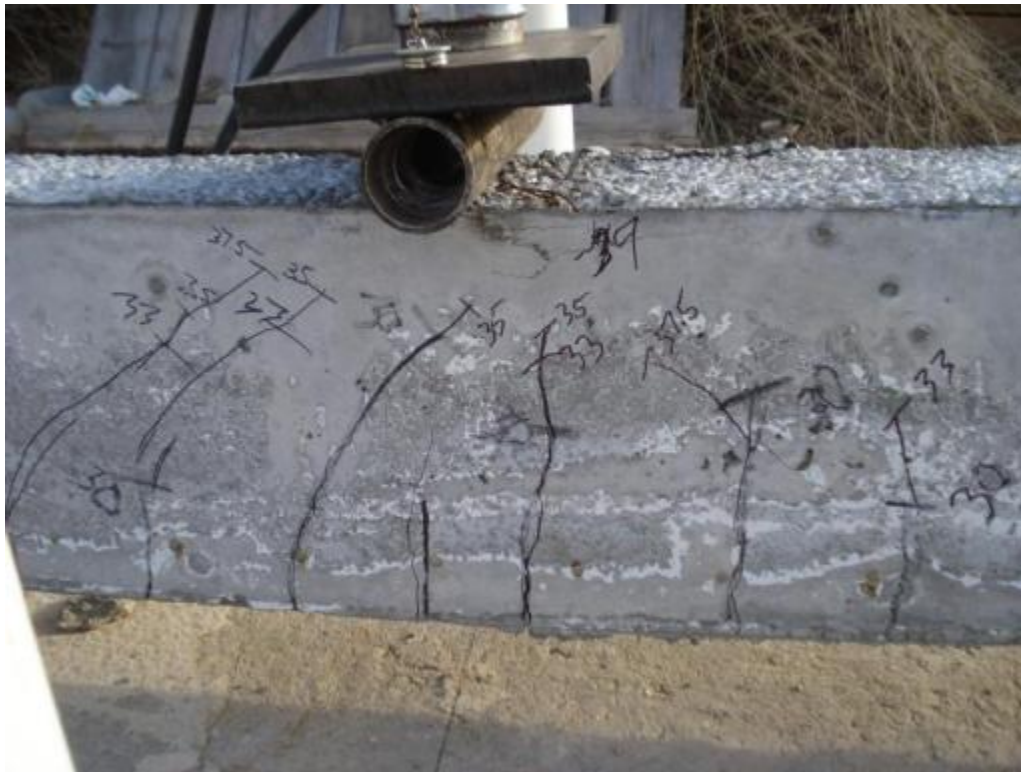
Figure 6.13: Cracking behavior of specimen NSC-4D
