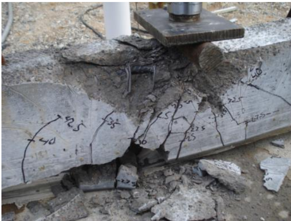
Figure 6.73: Cracking and failure of specimen HSS-2D
