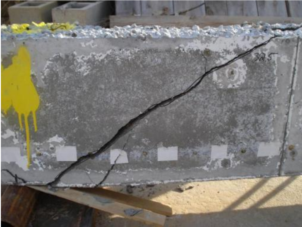
Figure 6.9: Shear cracking of specimen NSC-3D
