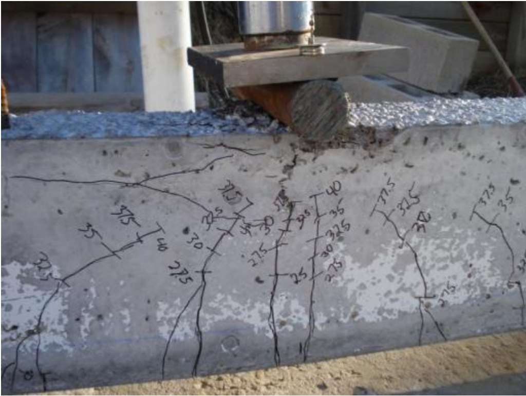
Figure 6.7: Cracking pattern of specimen NSC-2L
