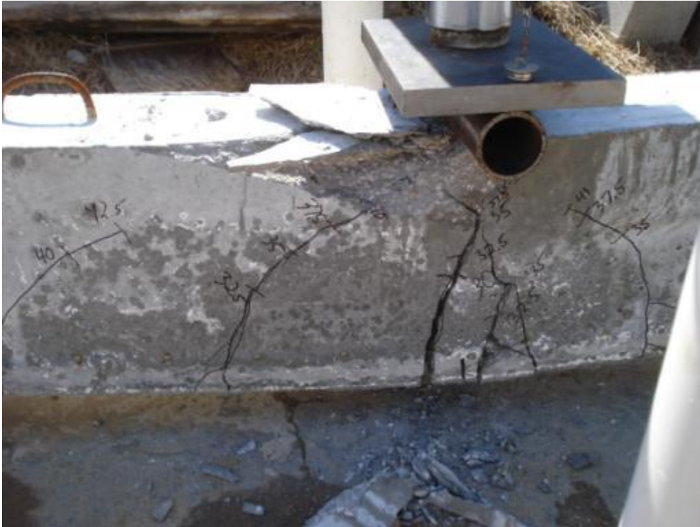
Figure 6.43: Cracking of specimen NSL-2L
