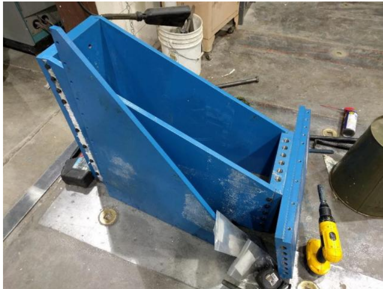
Figure 15 – Specimen cage being dry fit to check tolerances.
