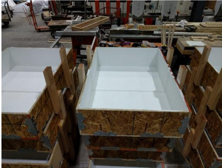
Figure 27 - Assembled and painted formwork without upper brace. Seventeen forms were built in total.
