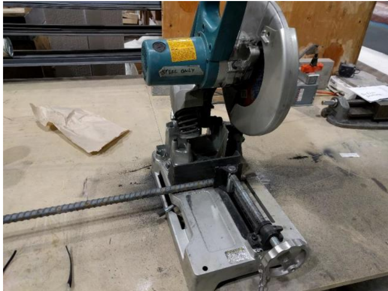
Figure 22 - Cutting reinforcing bar
