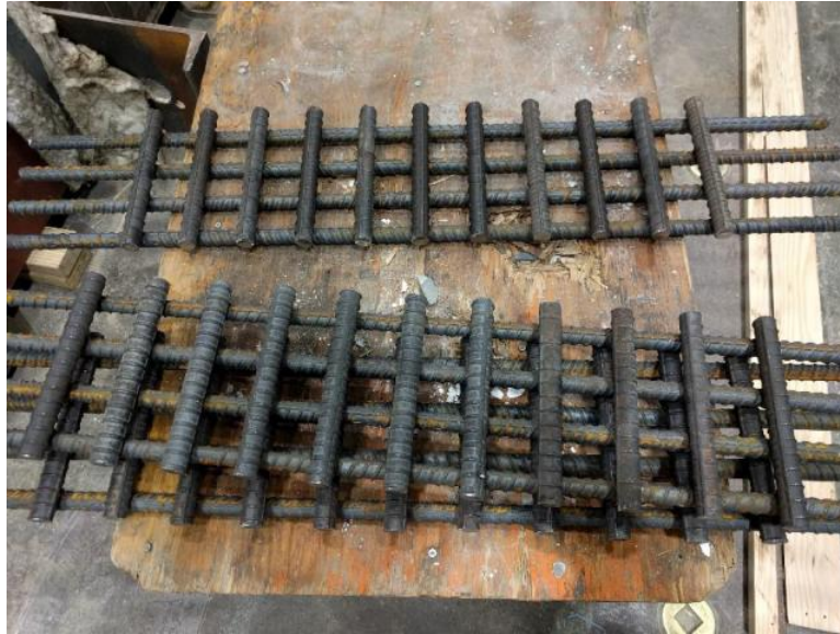
Figure 24 - Rebar cages ready to be welded to sample end plates.
