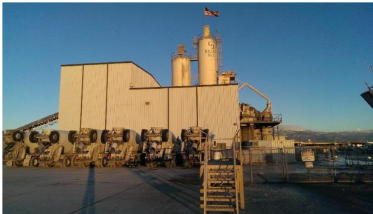
Figure 36 - Grand Junction Ready Mix, Grand Junction, Colorado
