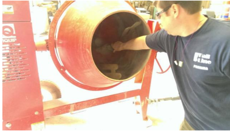
Figure 74 - Buttering the mixer
