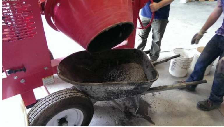
Figure 78 - Discharging freshly-mixed concrete
