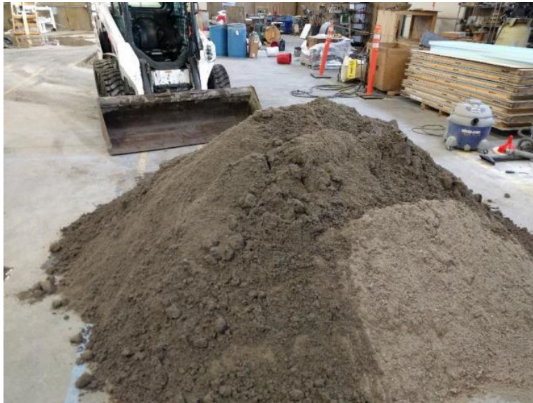
Figure 31 - Mixing fine aggregate and forming into pile.
