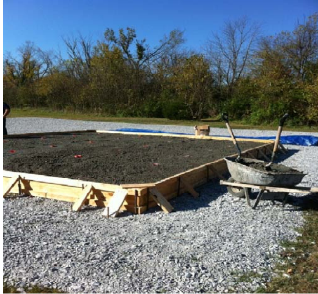
Figure 5.3: 24' x 20' 10" thick concrete base mat (Osweiler, 2012)
