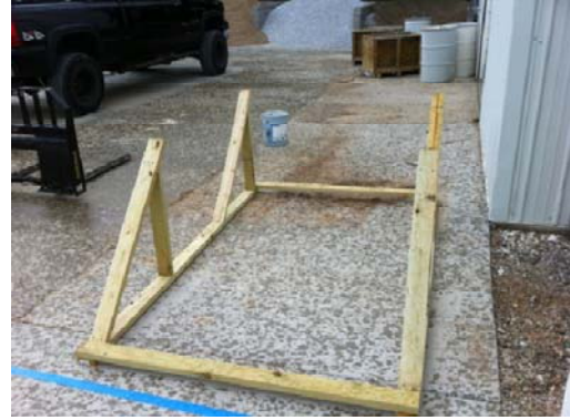
Figure 4.3: Front view of solar panel supports (Osweiler, 2012)
