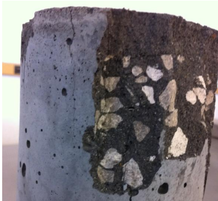
Figure 6.13: Segregation of aggregate and cement paste (Osweiler, 2012)
