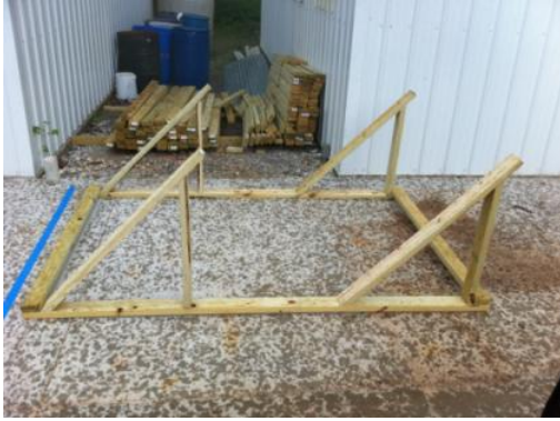
Figure 4.2: Side view of solar panel supports (Osweiler, 2012)
