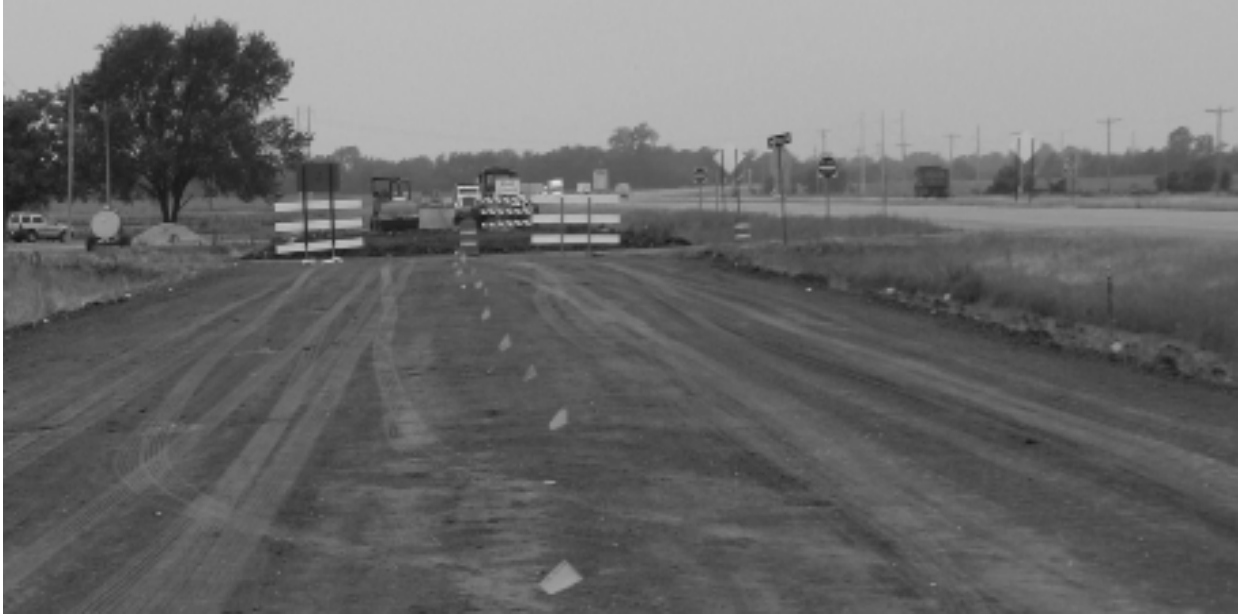
Figure 3.10. Finished cut subgrade (Howard 2006).
