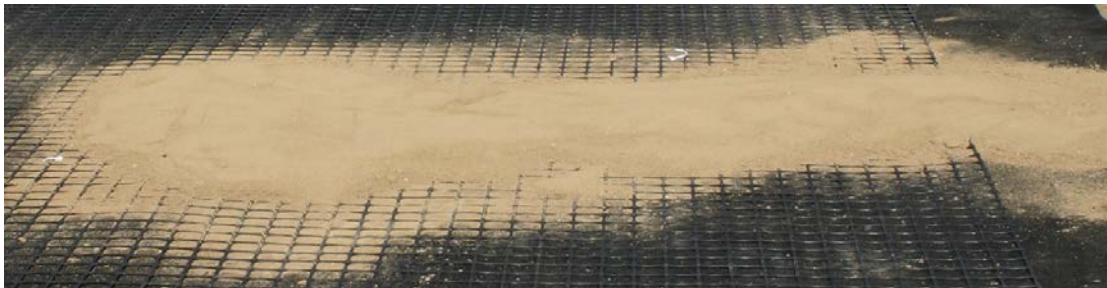
Figure 3.15. Sand covering geosynthetic strain gage and cable (Howard 2006).
