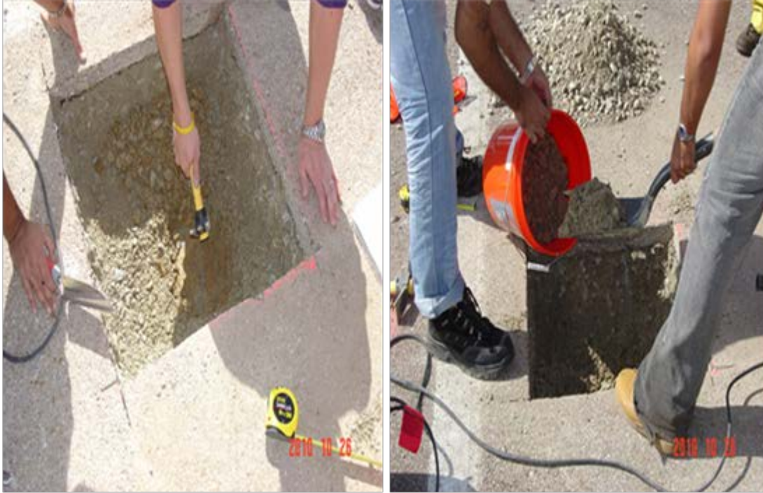
Figure 6.7. Base layer excavation and sampling at Section 2.
