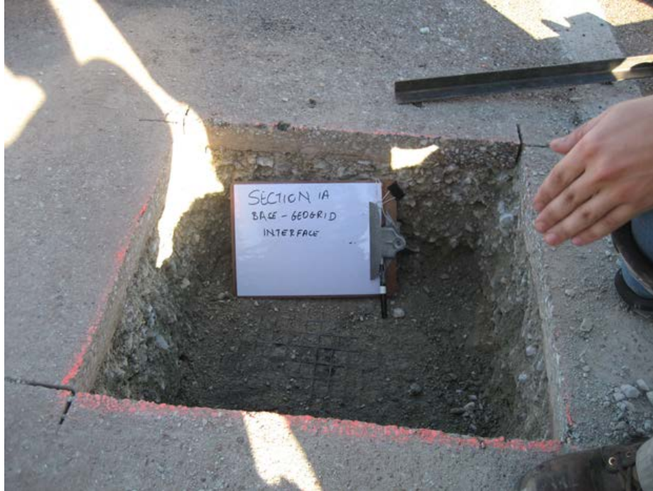
Figure 6.9. Subgrade-geosynthetic interface of Section 1A (Mirafi geogrid).
