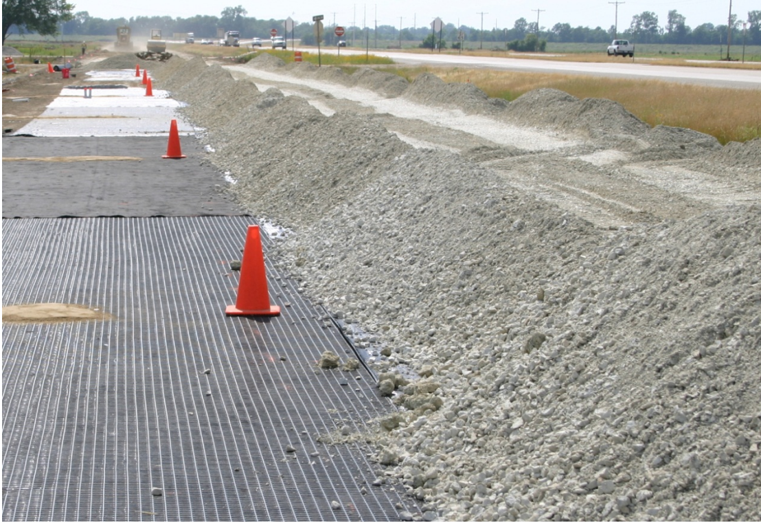
Figure 3.17. Base course placement on non-instrumented lane (Howard 2006).
