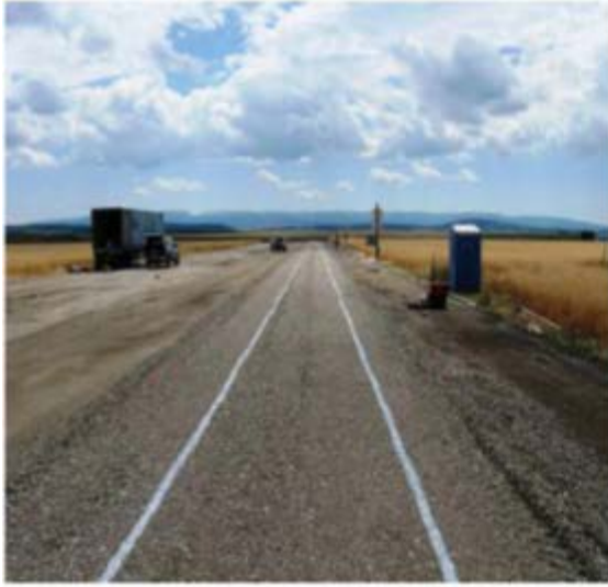
Figure 2.6. Full-scale field testing (Cuelho and Perkins 2009).
