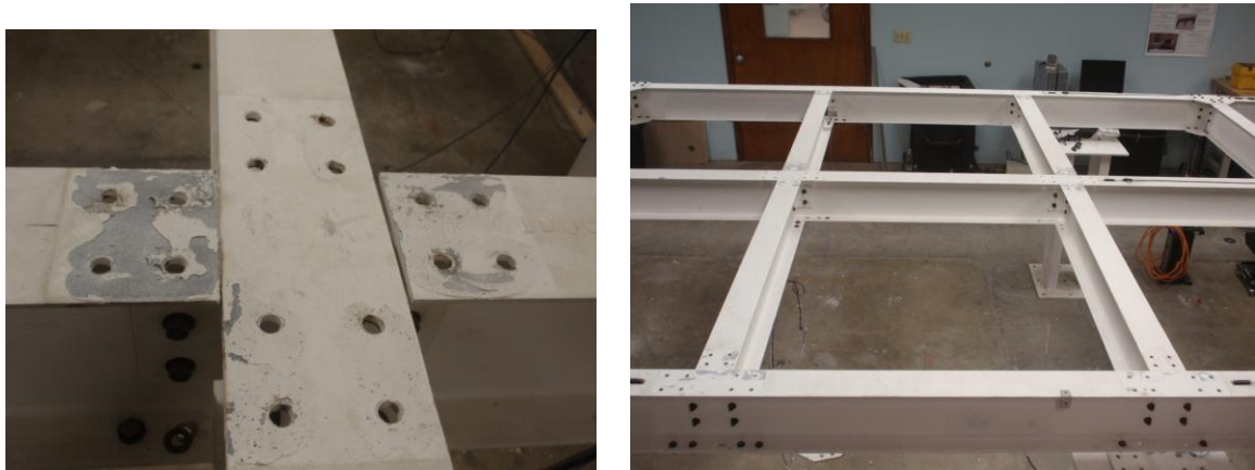
Figure 6.22: Damage Case #3 – Removal of Gusset Plates
