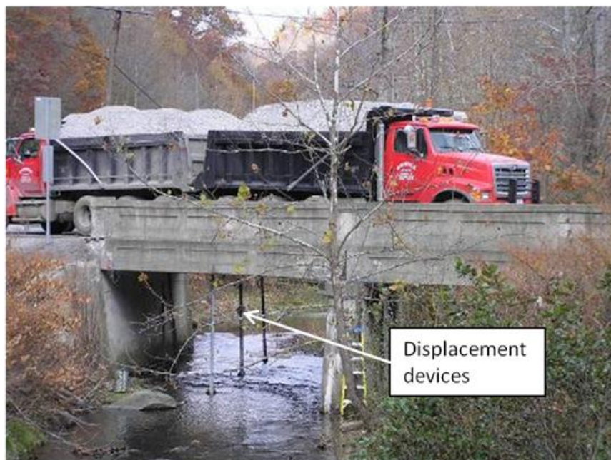
Figure 1.2: Static Bridge Testing
