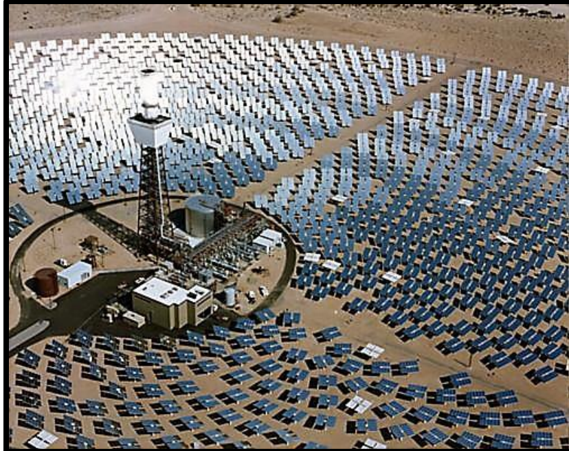
Figure 19: Central Receiver and Thermocline Tank at 10 MW Solar One in Daggett, CA (Morris, 2011)
