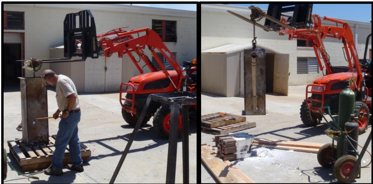
Figure 68: Heating Frozen Thermocline Test Chamber (Left) and Cleared Thermocline Chamber with Concrete/Salt Blockage on the Ground (Right)
