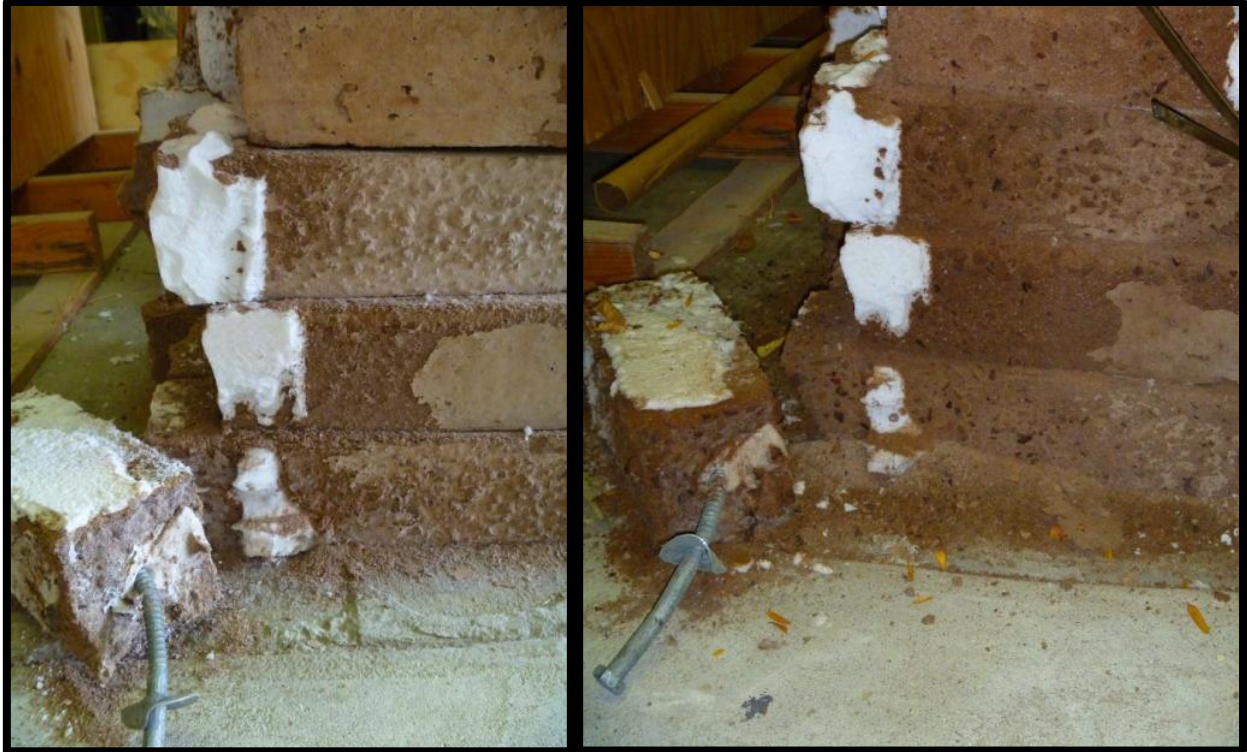
Figure 71: Progressive Deterioration of Mix 11 Specimens: 1 Month After Testing (Left) and 3 Months After Testing (Right)
