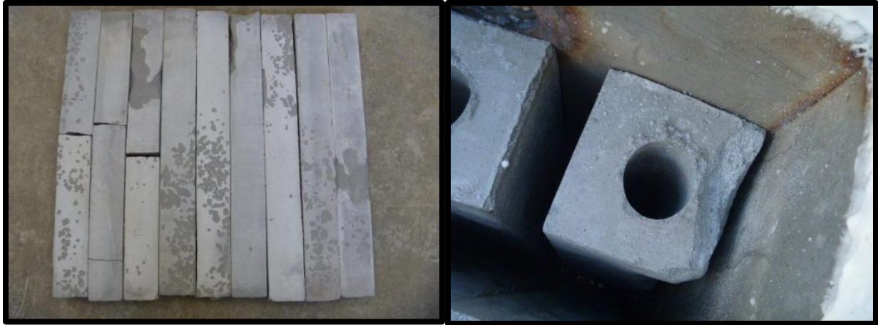
Figure 70: Spalling Damage to TC1000 Concrete Specimens
