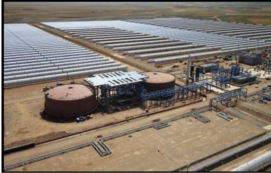
Figure 20: Two-Tank TES and Trough Array at 50 MW Andasol I in Grenada, Spain (Craig, 2011)
