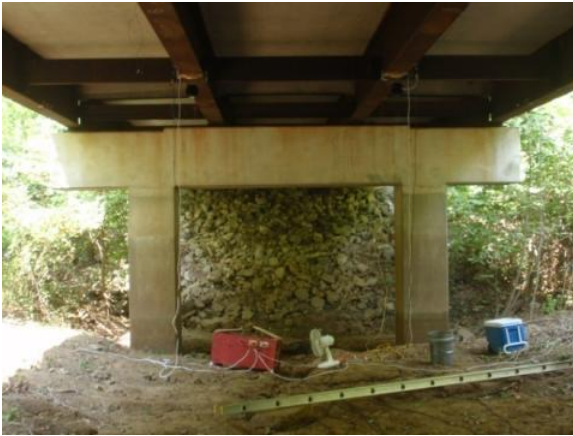
Figure 7.2. Photographs showing typical pier (left) and typical abutment (right). (Photos by EVF, Fayetteville, 10/18/13)
