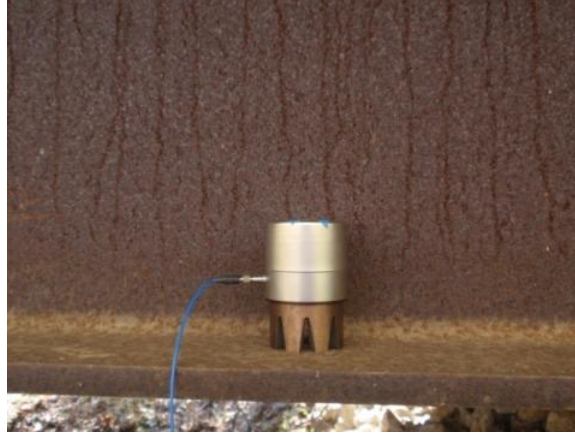
Figure 7.17. Photograph of typical accelerometer installation. (Photo by EVF, Fayetteville, 10/18/13)
