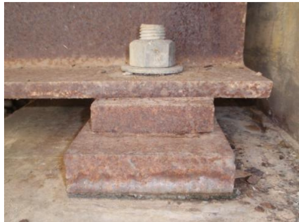
Figure 7.3. Photographs showing typical fixed bearing (left) and expansion bearing (right). (Photos by EVF, Fayetteville, 10/18/13)
