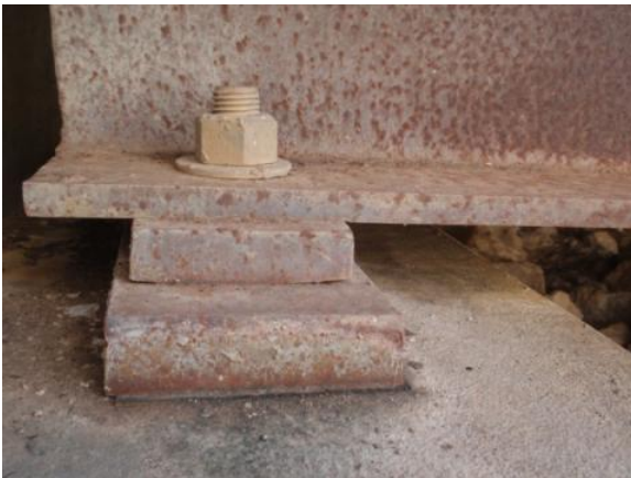
Figure 7.3. Photographs showing typical fixed bearing (left) and expansion bearing (right). (Photos by EVF, Fayetteville, 10/18/13)
