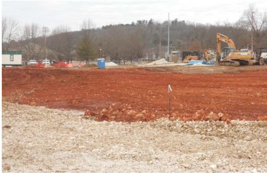
Figure 4.14. Example of a construction site near the Lot 56B infiltration sampling site. Topsoil has been removed and non-native soils have been introduced to the site and compacted.
