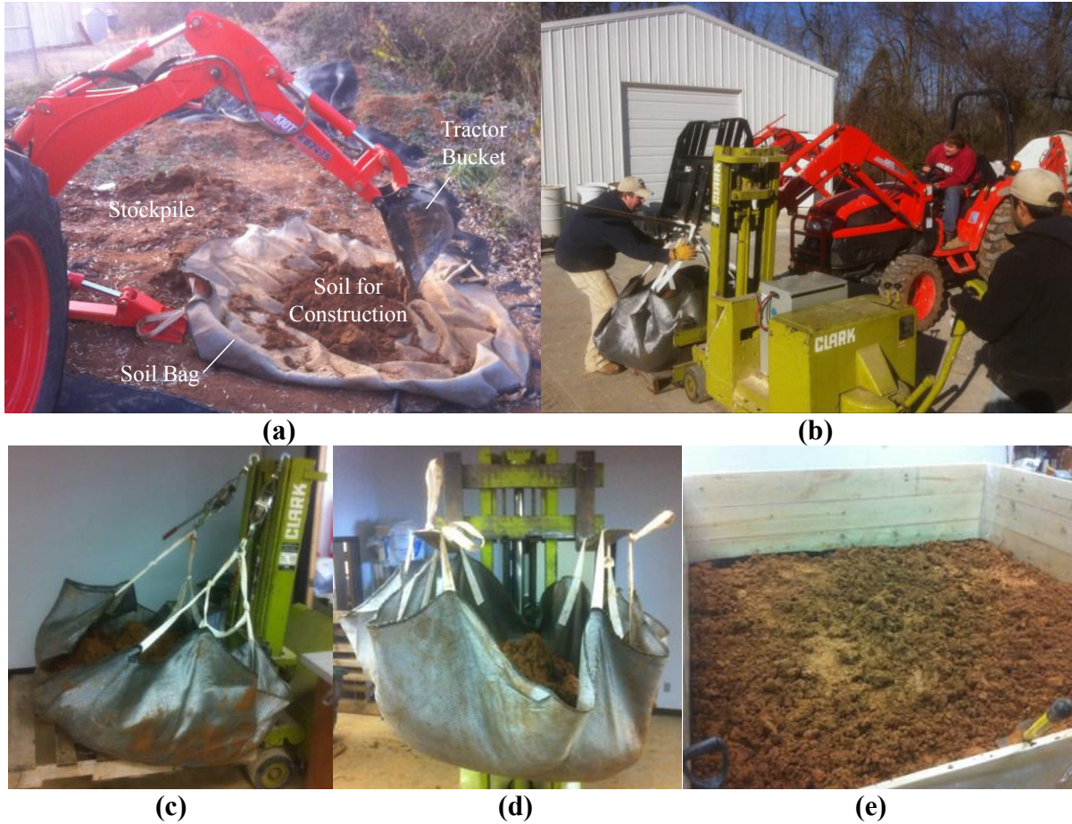
Figure 3.8. (a) Using the tractor to fill a bag with soil from stockpile, (b) filled soil bag being transferred from the tractor to the forklift, (c) soil bag being brought into the ERC using the forklift, (d) soil bag picked up using the forklift to place inside the test pad box, and (e) loose lift of soil in test pad box.
