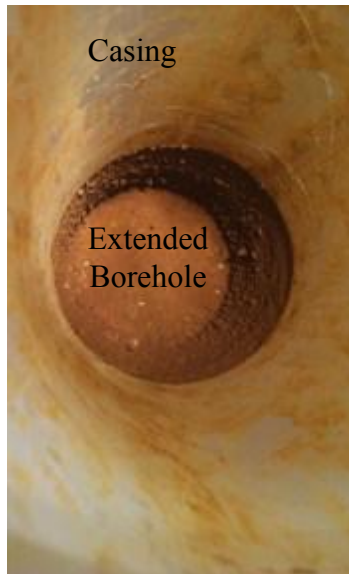
Figure 3.19. Photo of extended borehole.
