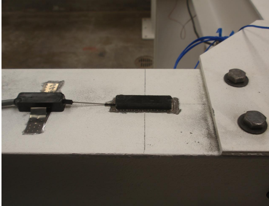
Figure 3.16: 350 Ohm weldable strain gage installed on grid model structure. Photo taken by Jason Herrman, Fall 2010 Engineering Research Center
