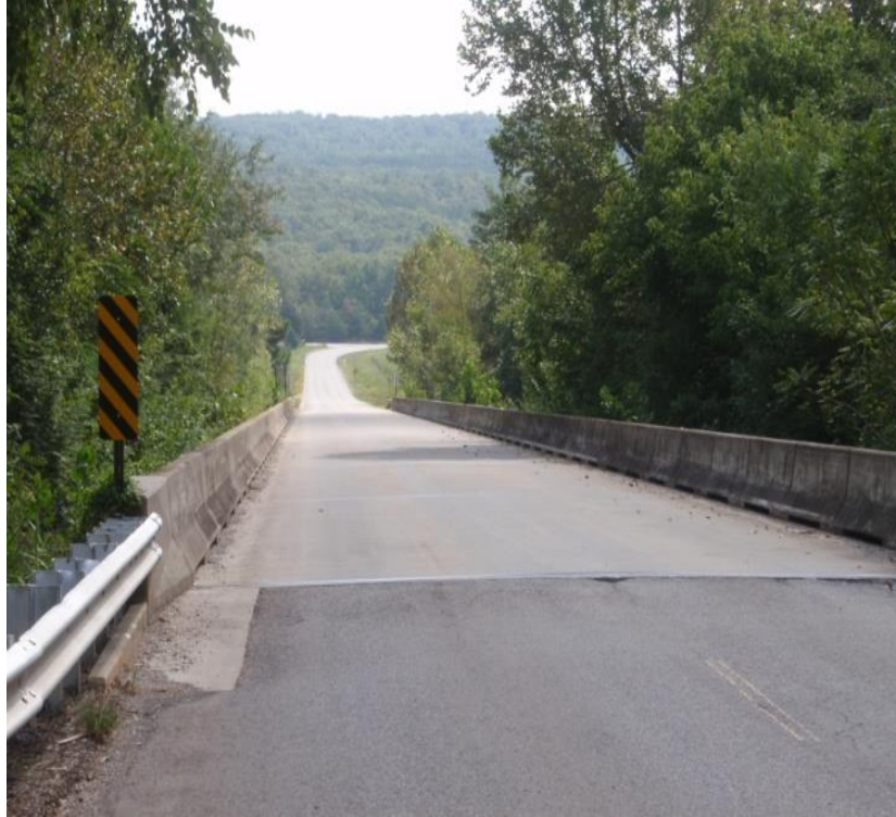
Figure 4.1: Hancil "Tiny" Hartbarger Bridge - concrete deck on multi-beam bridge. Photo taken by Jeremy Rawn, Fall 2010 Fayetteville, Arkansas
