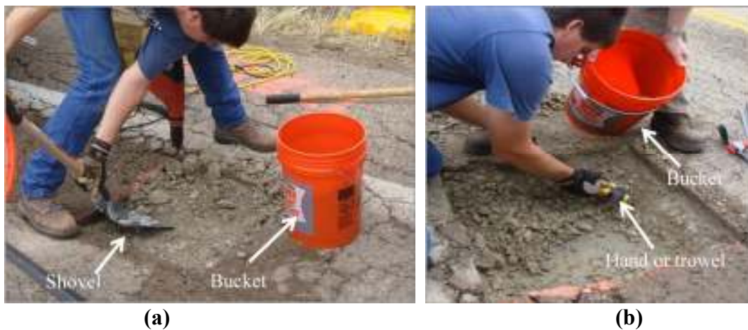
Figure 3.11. a) Shoveling and b) hand scooping base course samples into buckets.
