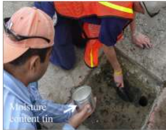
Figure 3.18. Subgrade moisture content sample.
