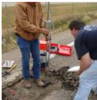
Figure 3.7. Dynamic Cone Penetrometer (DCP) testing in progress.
