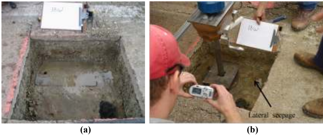
Figure 4.35. Lateral seepage observed in subgrade of Section 13W a) after DCP testing and b) after completion of CBR testing.
