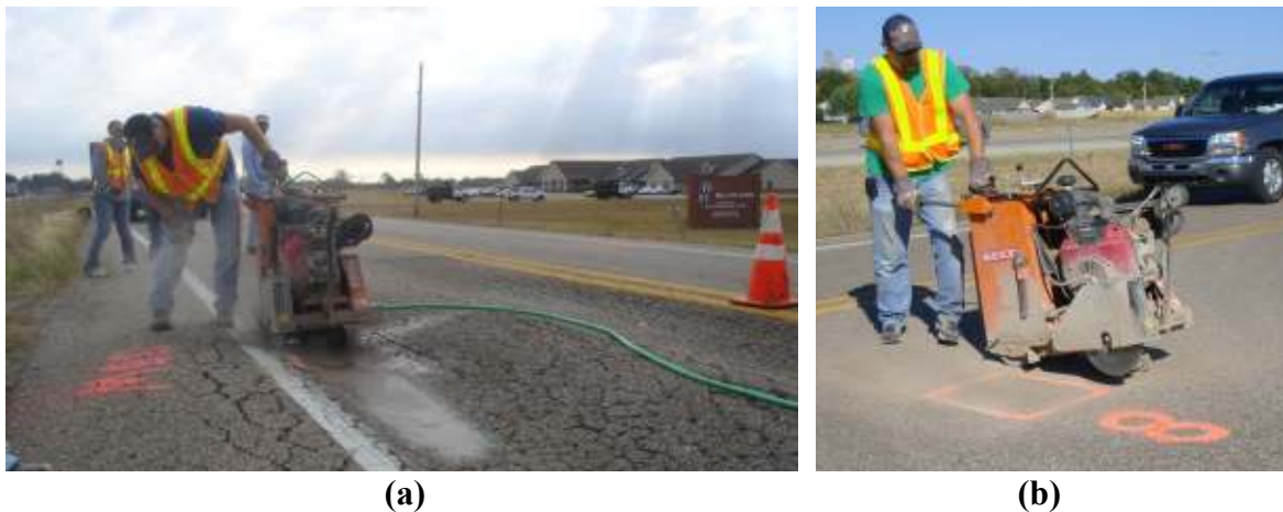
Figure 3.3. Two foot by two foot test sections cut by Arkansas State Highway and Transportation Department (AHTD) personnel using a wet concrete saw a) Section 13W and b) Section 8.
