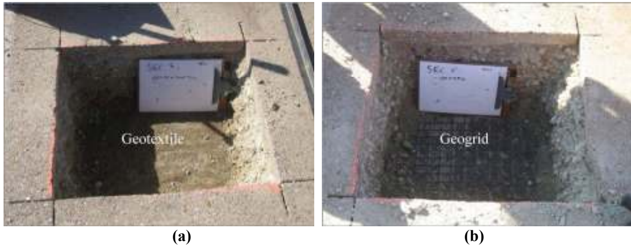
Figure 3.14. a) Typical geotextile/subgrade interface (Section 4) and b) typical geogrid/subgrade interface (Section 5).
